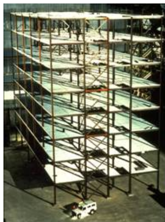
(a) Full-scale building tested in Cardington
