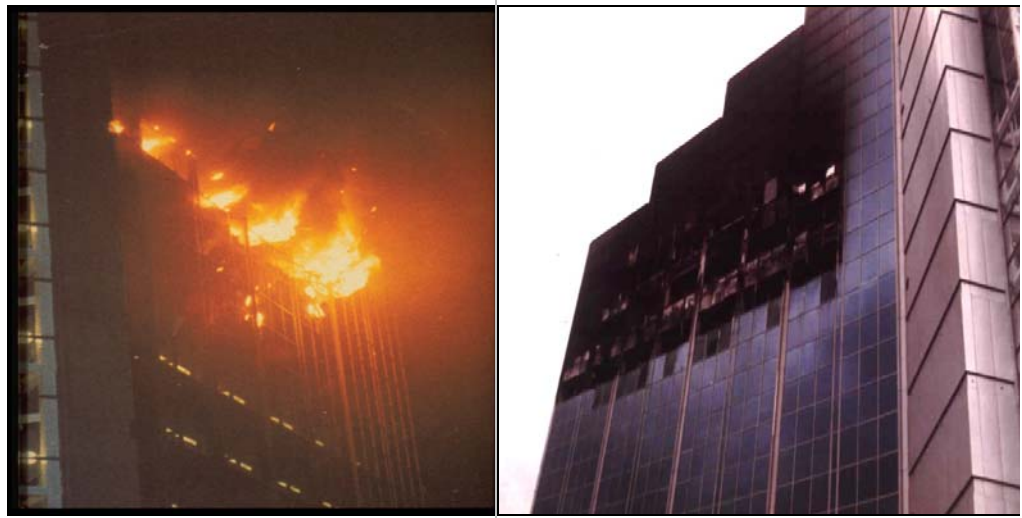
Figure 1.1 Fires in multi-storey buildings
