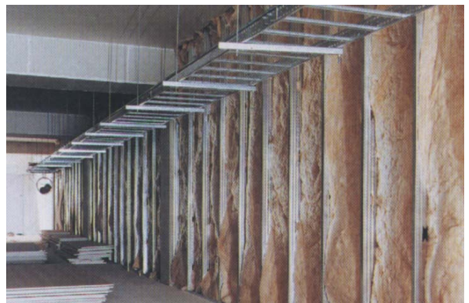
Acoustic insulation between the wall studs.
