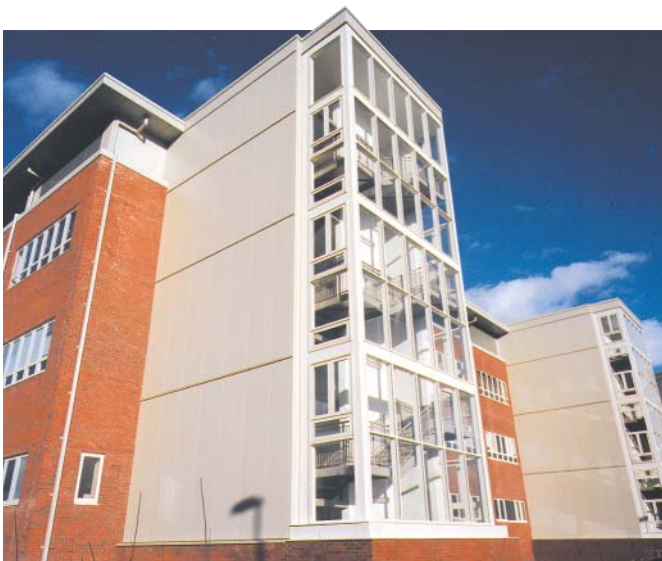
Infill walls used in Cumberland Hospital.
