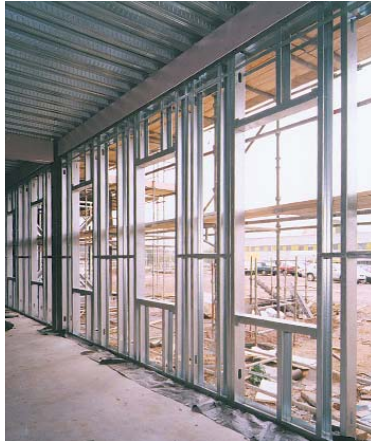
Infill walls used in Colchester Hospital.
