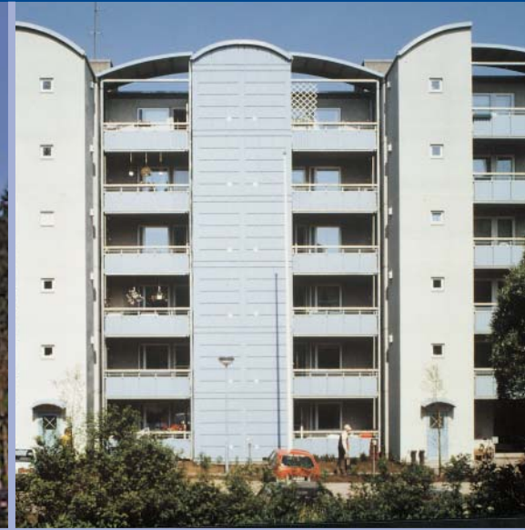
Pre-fabricated balconies and modular units at Forssa, Finland.
