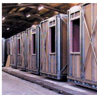
Modules fitted out at Unite.
