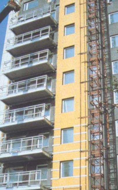
New balconies and over-cladding, Finland.
