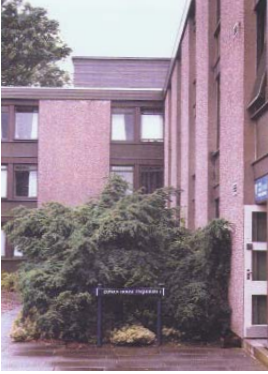
Original view of building.
