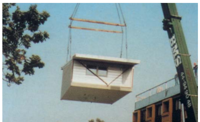
Modular roof-top units being lifted into place in the Copenhagen project.
