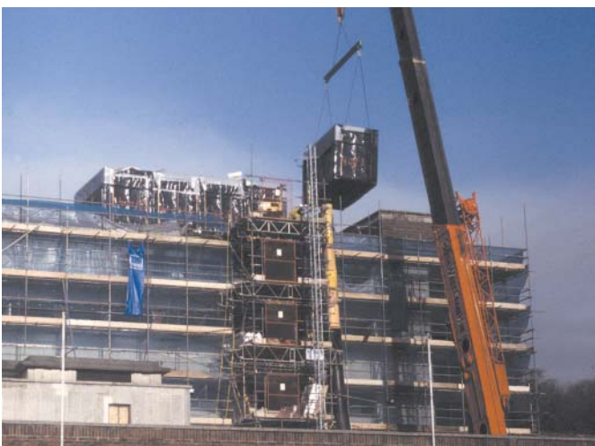
Roof top modules being lifted into place.
