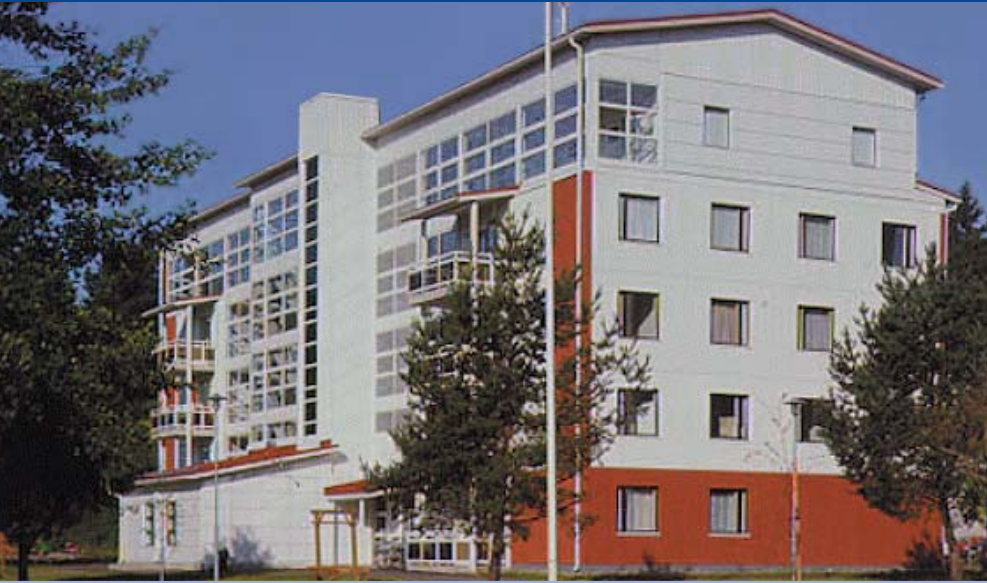
Roof-top apartments using modular units in Hämeenlinna, Finland.
