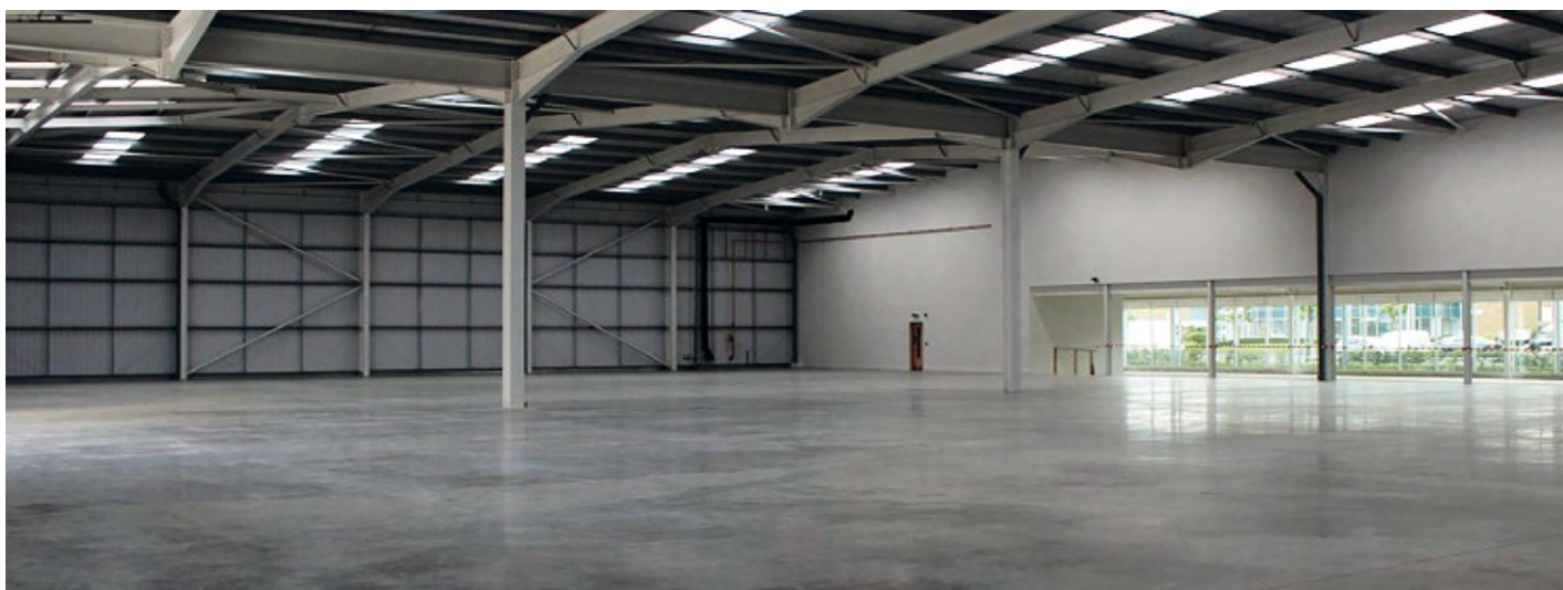
SEGRO warehouse and office building deconstructed and relocated on the Slough Trading estate in 2015
