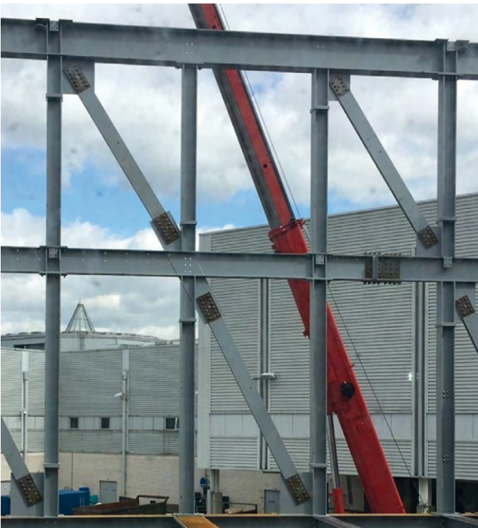
Figure 4.3: Thick end plate splices. Photo courtesy of H Young Structures Ltd
