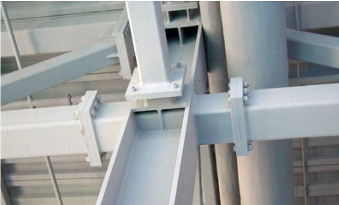
Figure 4.2: Thick end plate splices
