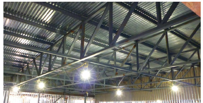
Figure 5.1: Top and bottom boom restraints
