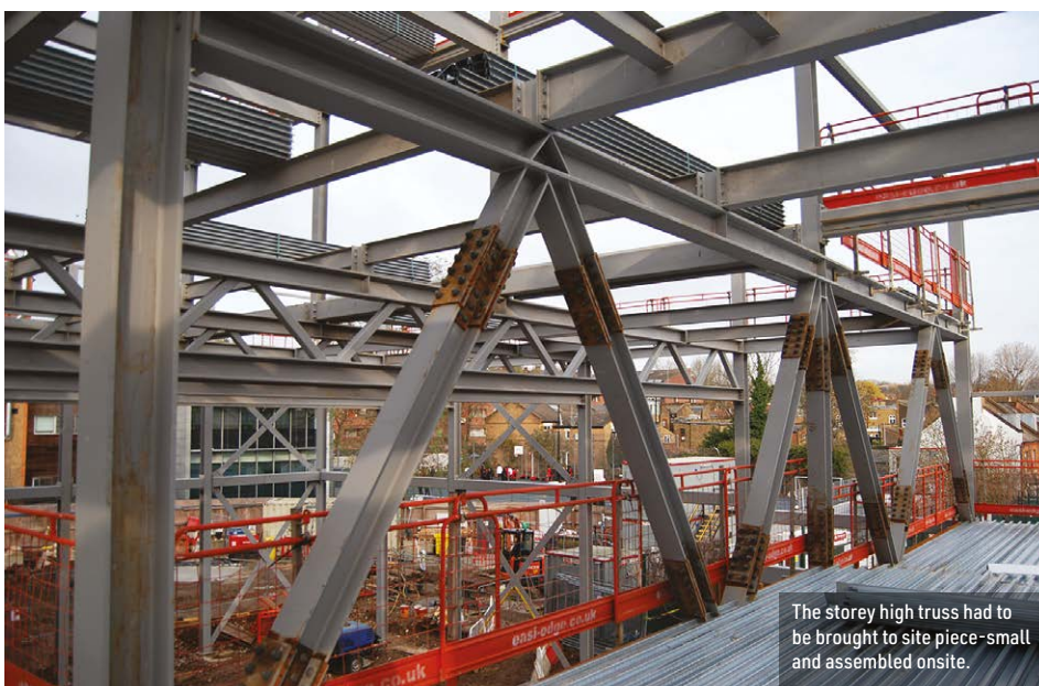
Four 16.6m-long x 1.4m-deep trusses span the main hall.
