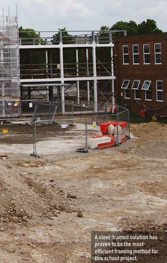
The sports hall is formed with a series of 19m-long rafters.
