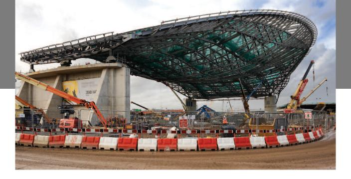
erection, it was necessary to install a temporary tie comprising eight high tensile steel bars between the north cores. This was pre-stressed before the roof was lifted off the temporary trestles.
