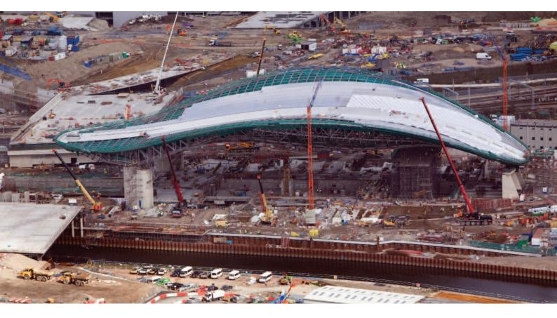
The London Aquatics Centre will mark the gateway to the 2012 Olympic Park. The stunning waveform shape of its complex steel roof sweeps dramatically upwards in a smooth curve from the south end and then down again over the northern cantilever, while the western and eastern tips curve upwards at the edges.
