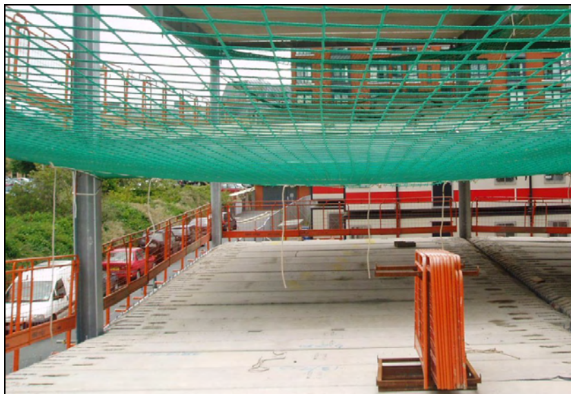
Figure 5.1 Edge protection and net fall arrest system
