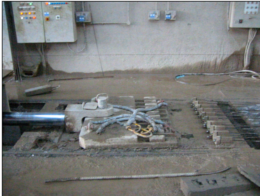
Figure 1.9 Wires being stressed
