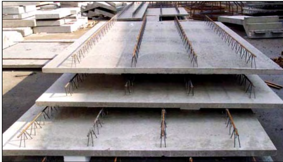
Figure 1.7 Precast lattice slab floor units
