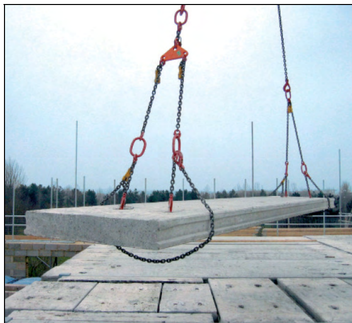
Figure 5.5 Lifting of units
