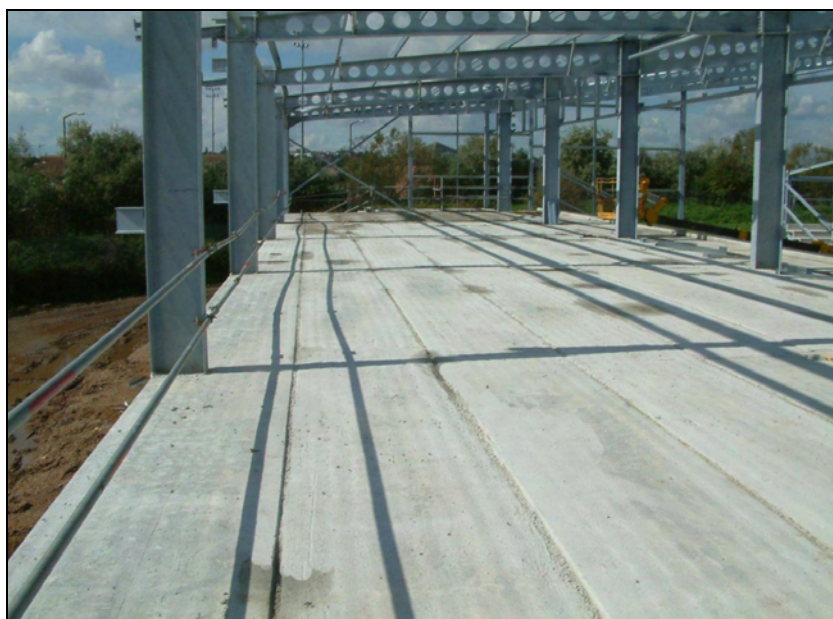
Figure A.14 Burton Albion stadium during construction
