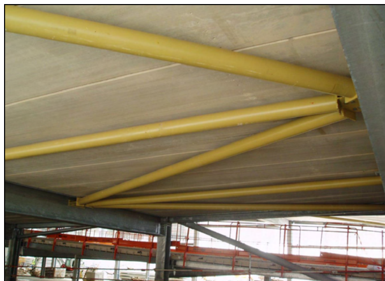
Figure 5.10 Temporary bracing for long span beams
