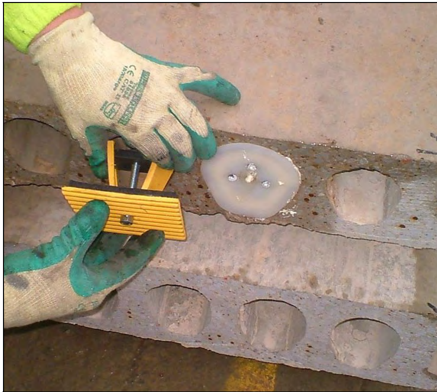
Figure 1.17 Hollow core end-sealing devices
