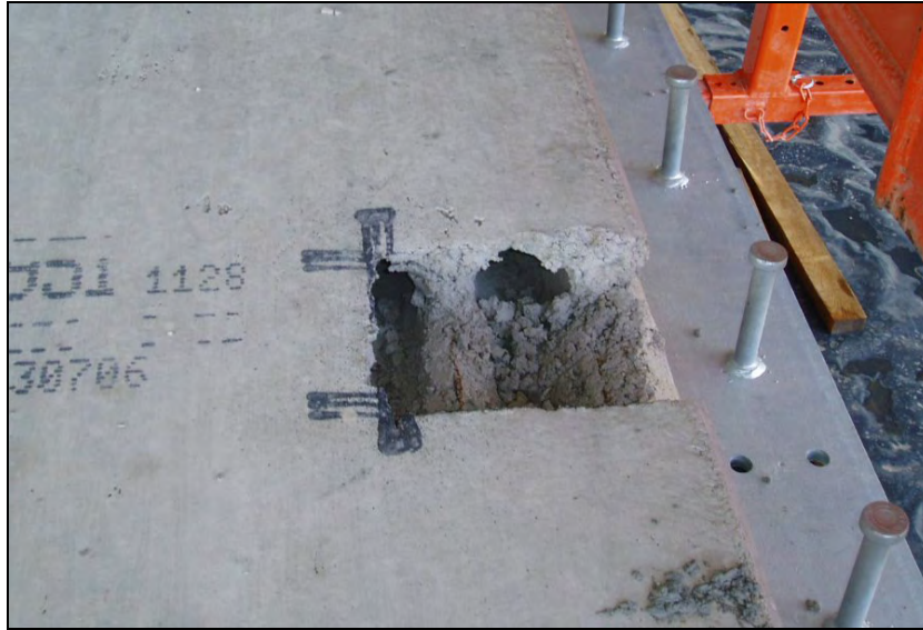
Figure 4.13 Side pocket in precast unit
