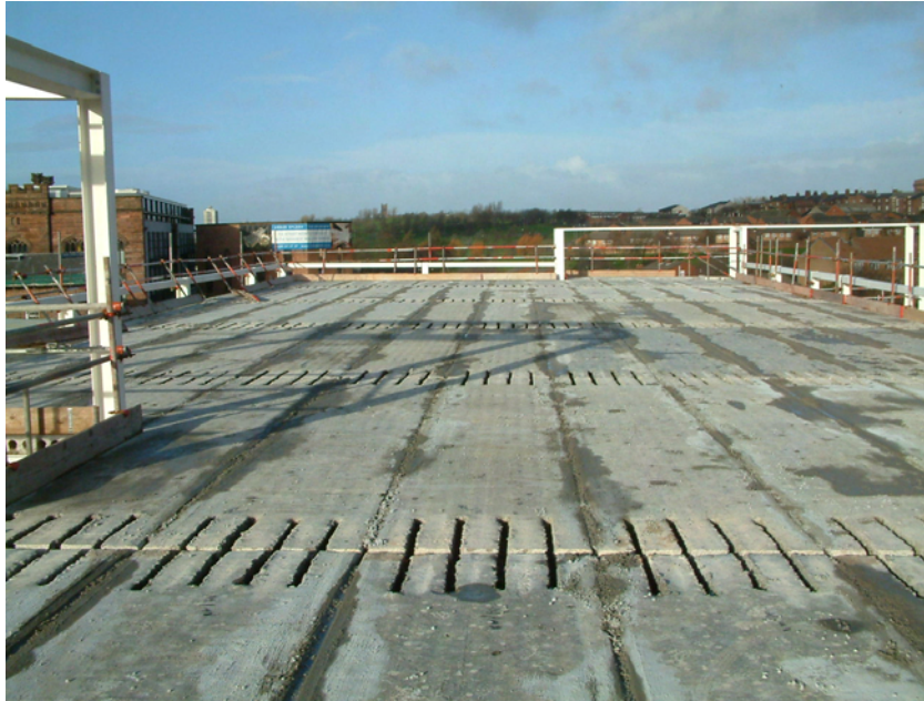
Figure A.11 Car park deck during construction
