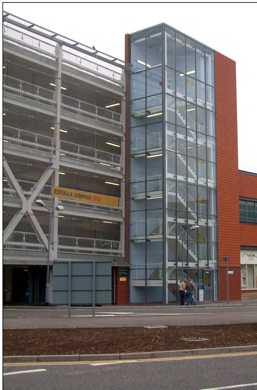
Figure A.10 Multi-storey car park, Nuneaton
