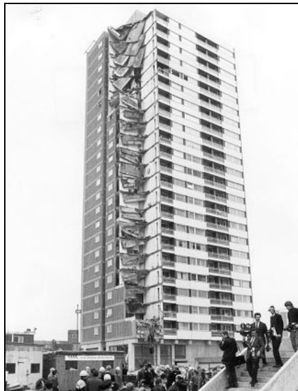
Figure 4.1 Partial collapse of Ronan Point (1968)
