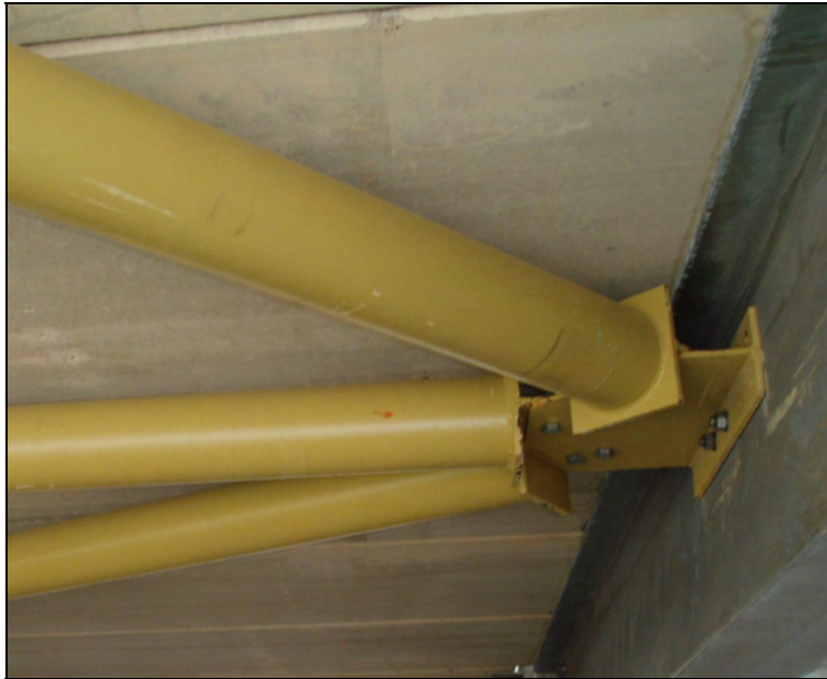
Figure 5.11 Temporary lateral restraint detail to compression flange
