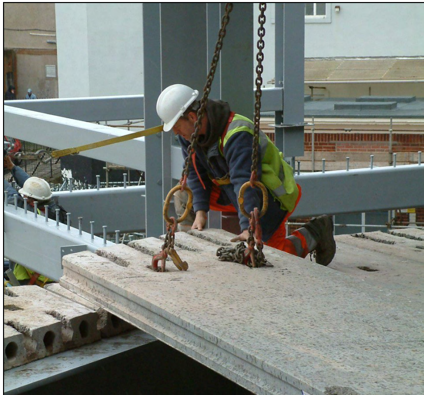
Figure A.9 Placing units during construction
