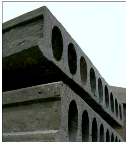
Figure 1.1 Hollow core floor units
