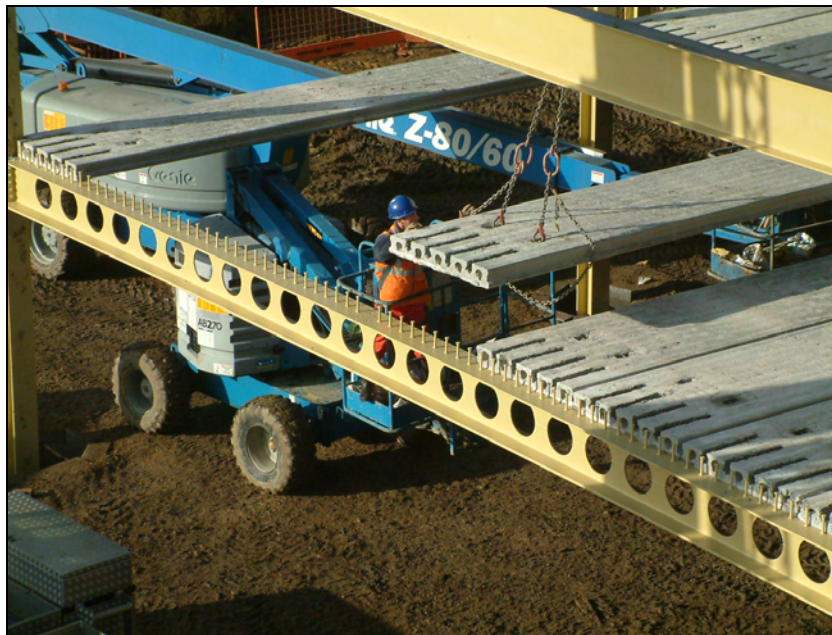
Figure A.5 Construction of the floor at Ikea, Manchester
