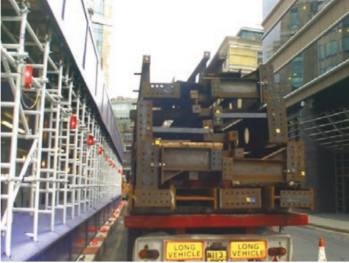
Load ready for unloading at a city centre site
