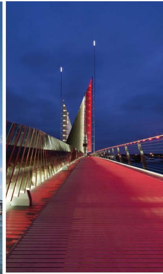
The 2.4m-wide walkways on either side of the bridge are separated from traffic by a stainless-steel screen that is designed in a wave form.
