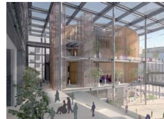
The atrium acts as the main visitor entrance for the civic centre. All of the slimline steelwork is visible and is an important aesthetic element of the 31m-high structure.
