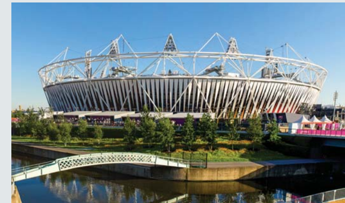
Some 2,500 of the 3,850 tonnes of steel tubing in the Olympic stadium's roof trusses was reclaimed from old gas pipes.
