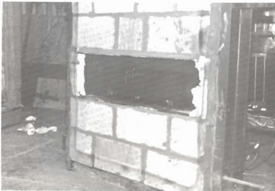
THE EXPOSED SIDE OF A PERIMETER BEAM SET IN THE WALL OF THE 1 m CUBE FURNACE (AFTER TESTING) FIG. 24(b)
