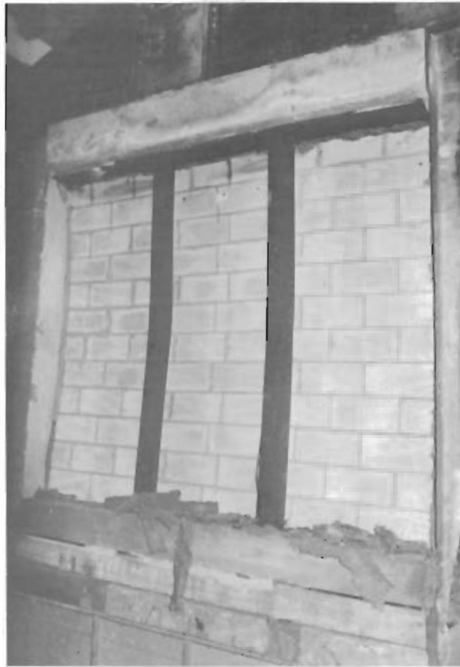
THE EXPOSED WALL SURFACE AFTER TESTING FIG. 19(d)
