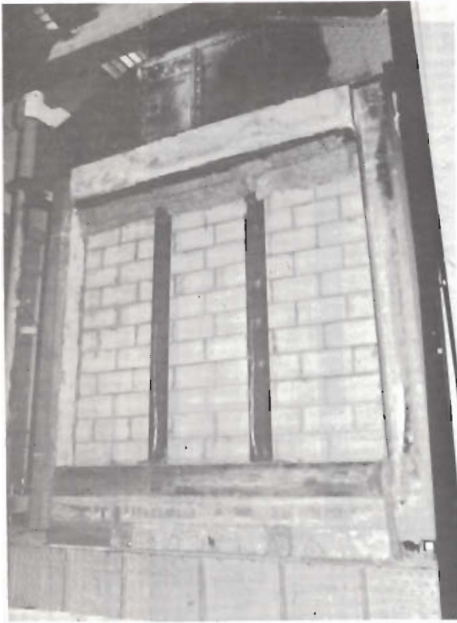
THE EXPOSED WALL SURFACE BEFORE TESTING FIG. 19(b)
