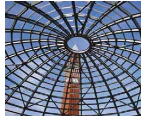
The dome contains more than 500 individual steel elements.
