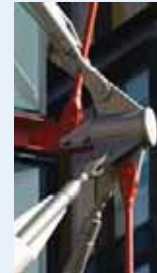
Quality of the exposed steel junctions was a priority.
