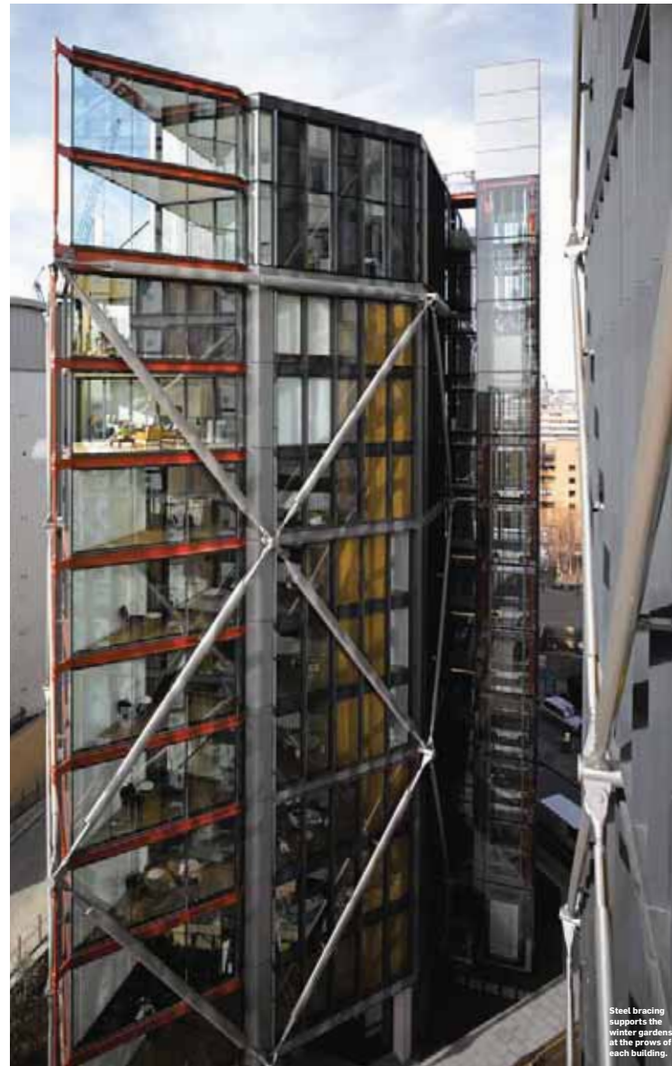
Red steel beams frame the inside of the lift hallways.
