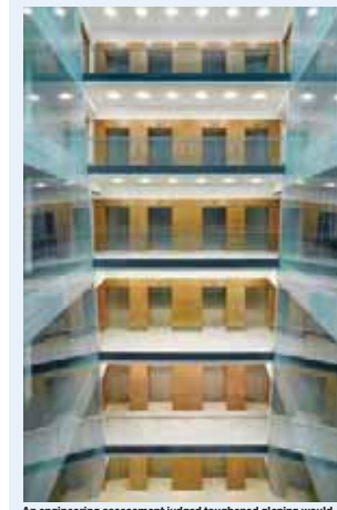
An engineering assessment judged toughened glazing would provide adequate fire protection in the atrium.
