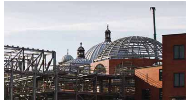
The steel dome and auditorium under construction, with the crescent's original domed buildings in the background.
