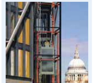
A lift core with St Paul's Cathedral in the background.
