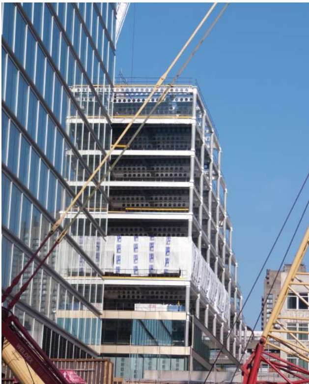
Figure 1-10: Moorgate Exchange, London (during construction)
