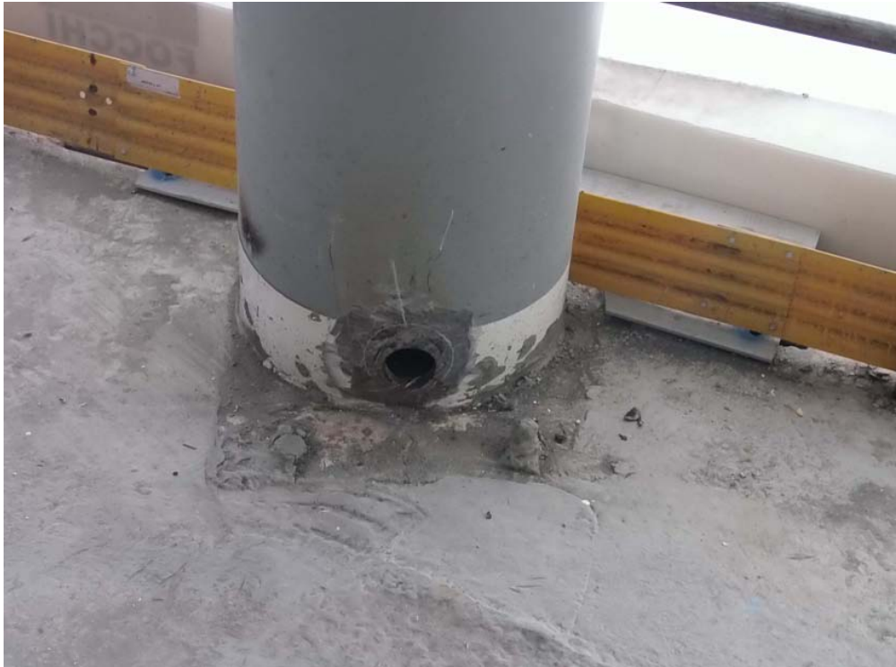
Figure 1-12: Concrete pumped into the column from base
