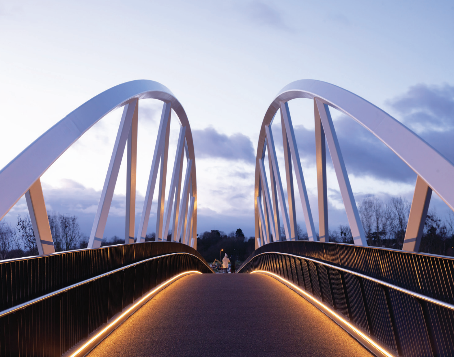
PICTURED: HAMS WAY FOOTBRIDGE PHOTOGRAPH: SIMON KENNEDY
