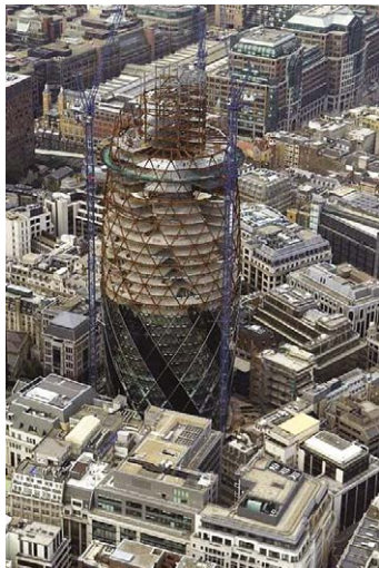
Figure 3: Swiss RE building showing work progressing up the building
