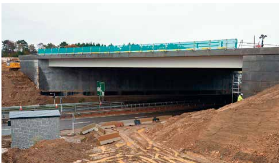
One of the 46m-long girders for the North Deeside Overbridge is delivered
