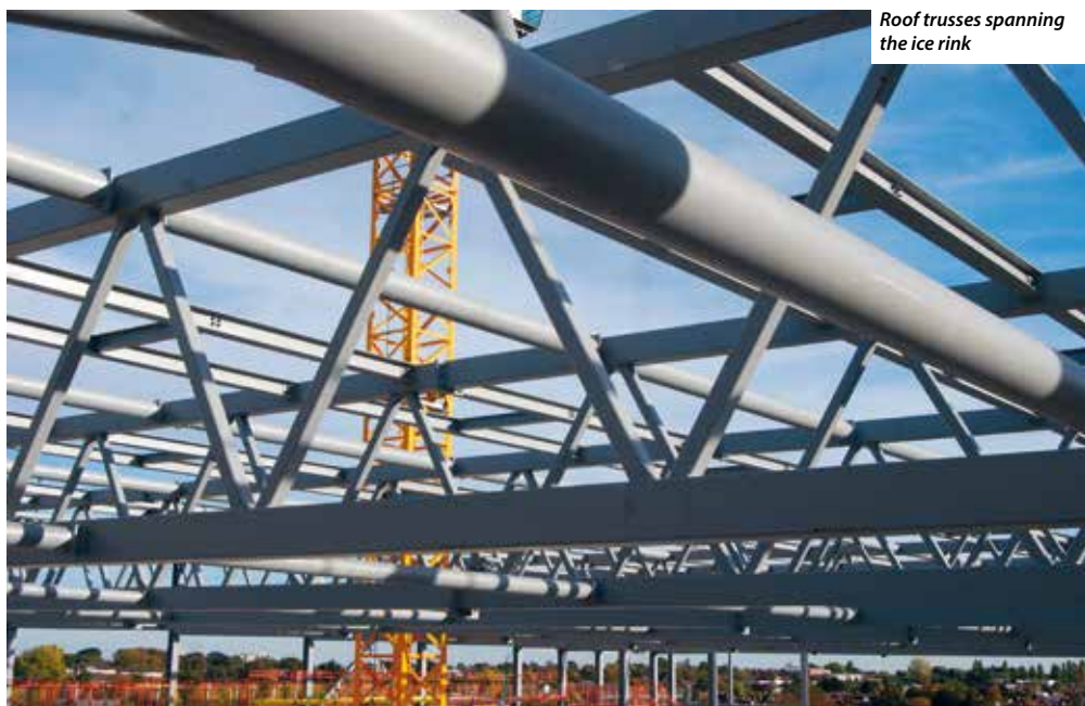
The upper-level ice rink under construction
