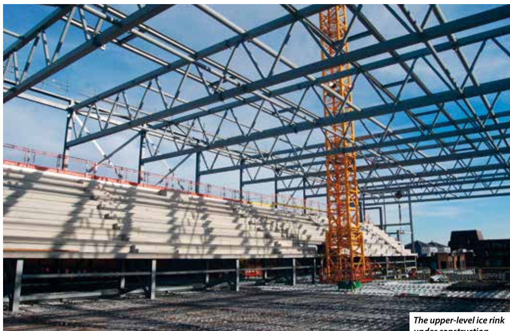
Roof trusses spanning the ice rink
