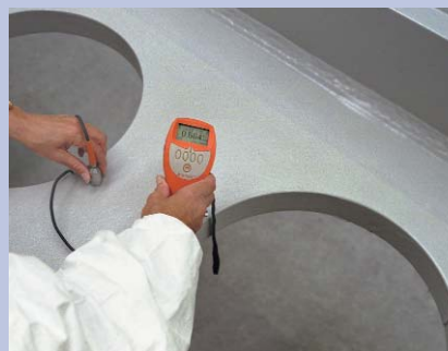
Intumescent coating being checked off-site.
