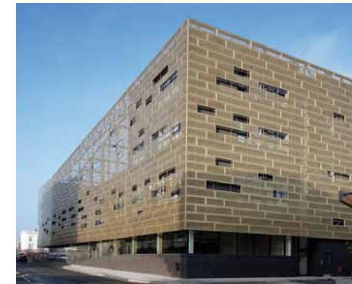
Distinctive copper cladding unites the multi-use Deptford Lounge.
