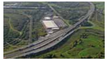
Repairs avoided a £100m viaduct rebuild.
