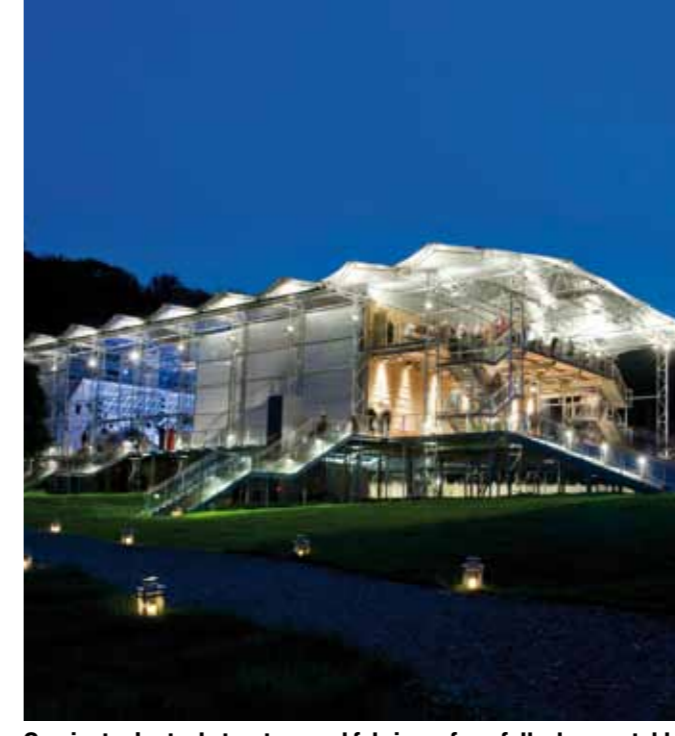
Garsington's steel structure and fabric roof are fully demountable.
