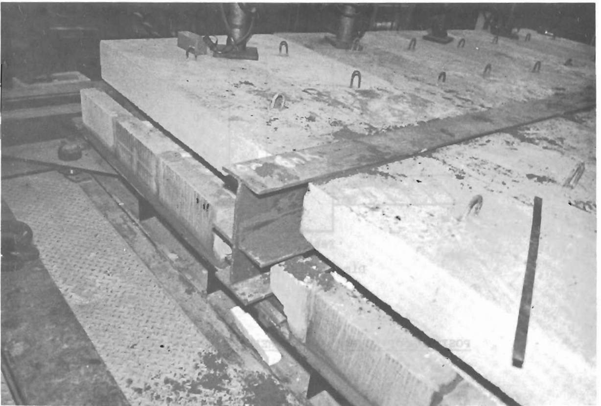
CONSTRUCTION OF TEST ARRANGEMENT
