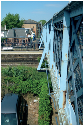
Figure 2: Bridges with external bracing to restrain the compression flange
