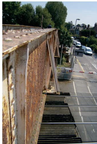
Figure 2: Bridges with external bracing to restrain the compression flange
