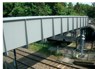
Figure 5: Footbridge with u-frames; cross section
