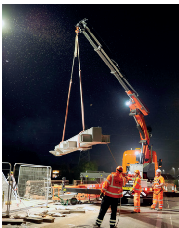
Figures 3 & 4: Countess Wear Footbridge: Left: Stainless steel cantilevers being lifted into position during a night closure; Right: Stainless steel parapet posts and handrails
