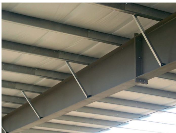
Figure 6: typical bracing to rafter
