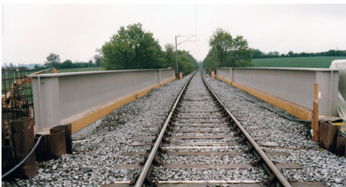
Figure 3: "Half-through" bridge
