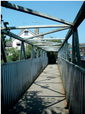
Figure 1: Truss bridge with bracing between the compression chords
