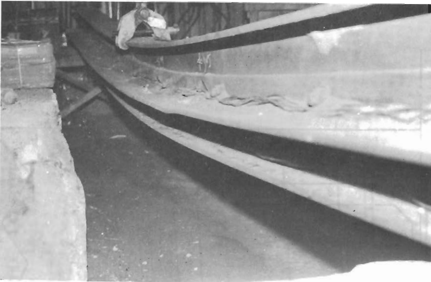
Uniform deflection of angle and beam (a)
