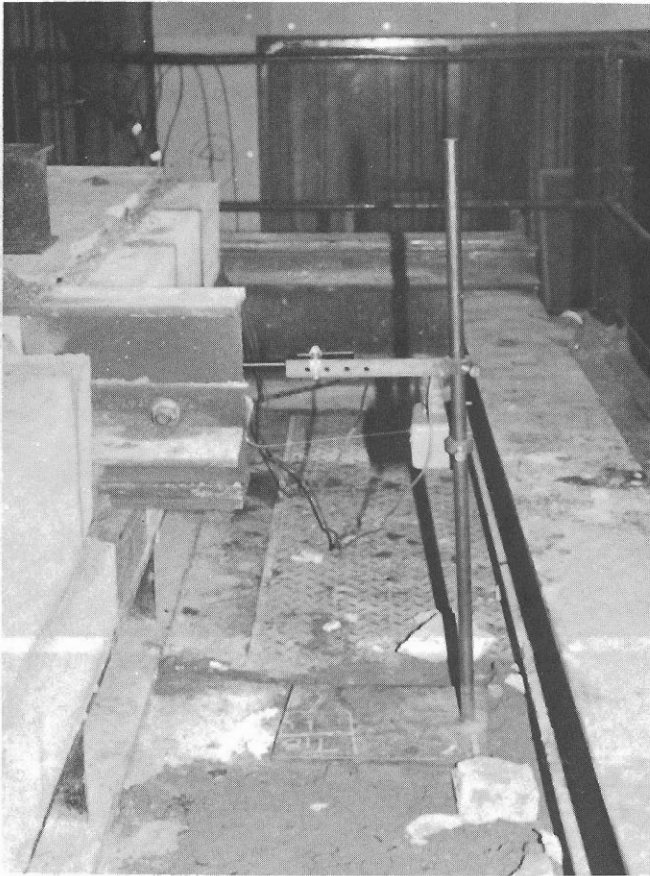
MONITORING BEAM END MOVEMENT
