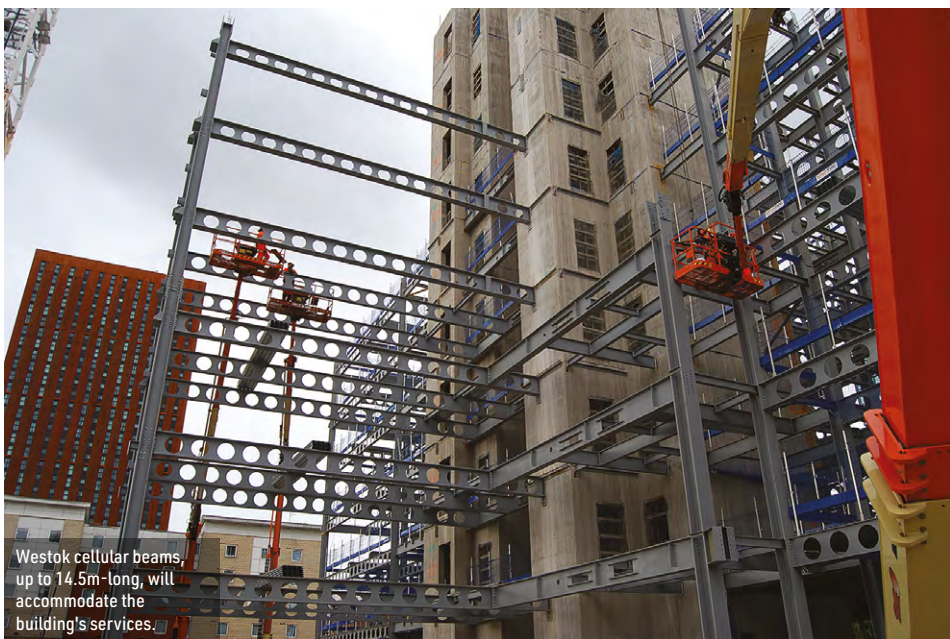
The steel frame gains its stability from a centrally-positioned concrete core.
