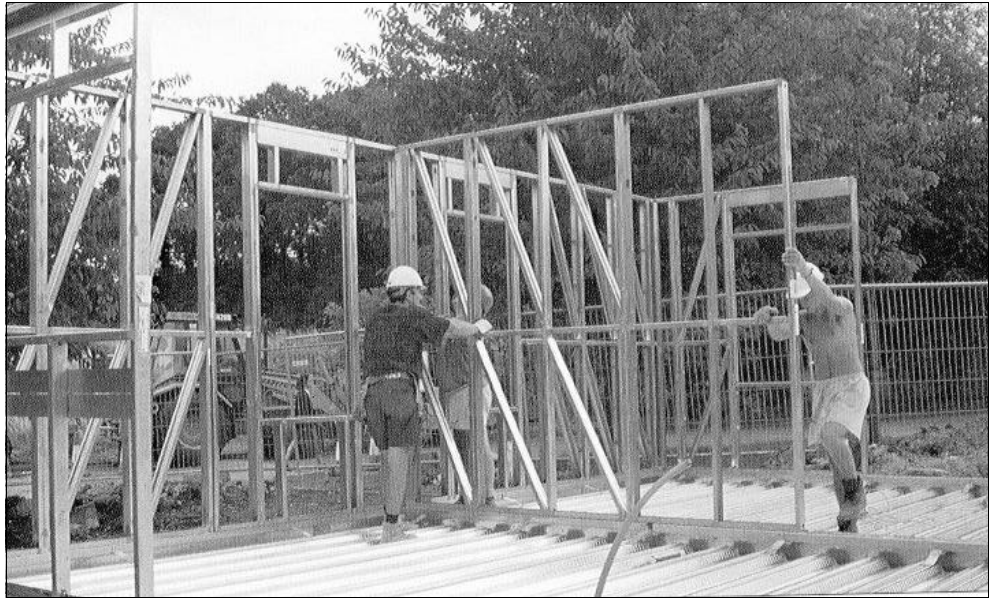
Figure 1.2 Light steel framing using prefabricated panels
