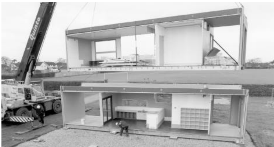
c) Open sided units used to form larger spaces (Portakabin Ltd)
