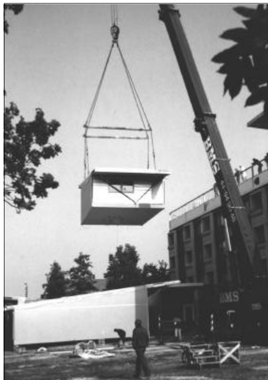
Figure 5.6 Modular over-roofing project in Copenhagen
