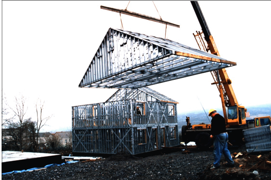
Figure 4.19 Pre-assembled roof structure craned onto a light steel framed house
