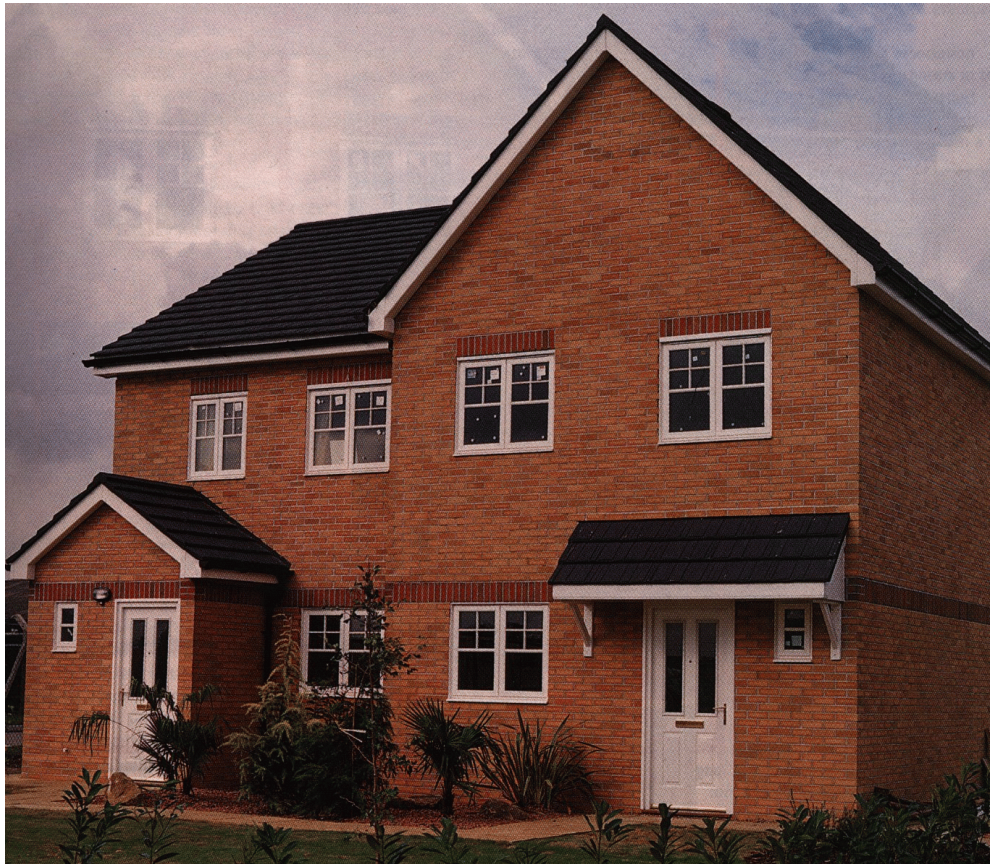
Figure 1.2 Semi-detached modular houses constructed by Britspace Ltd
