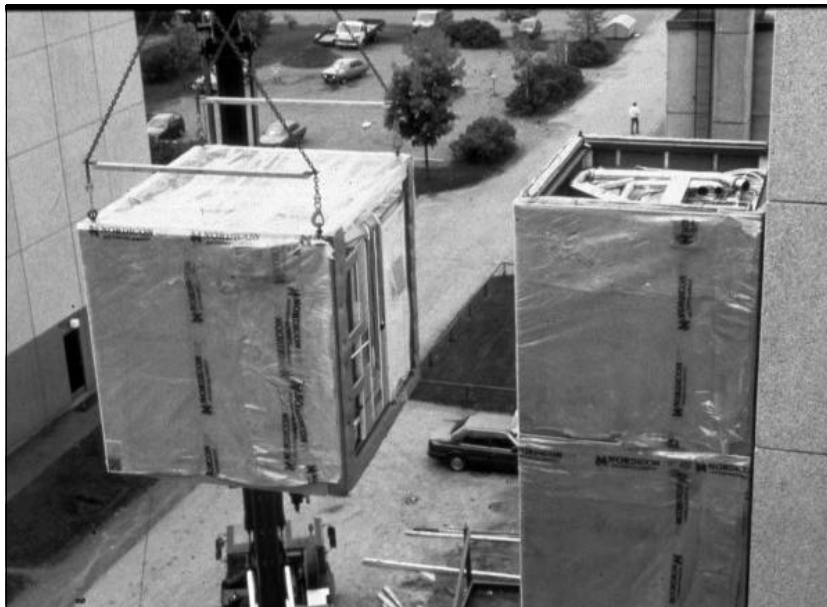
Figure 5.4 Lifting and installation of modular bathroom units
