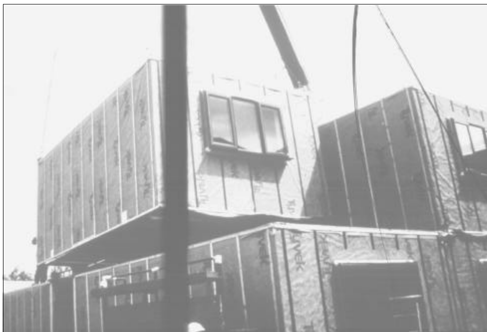
Figure 3.12 Installation of a module with its protective covering
