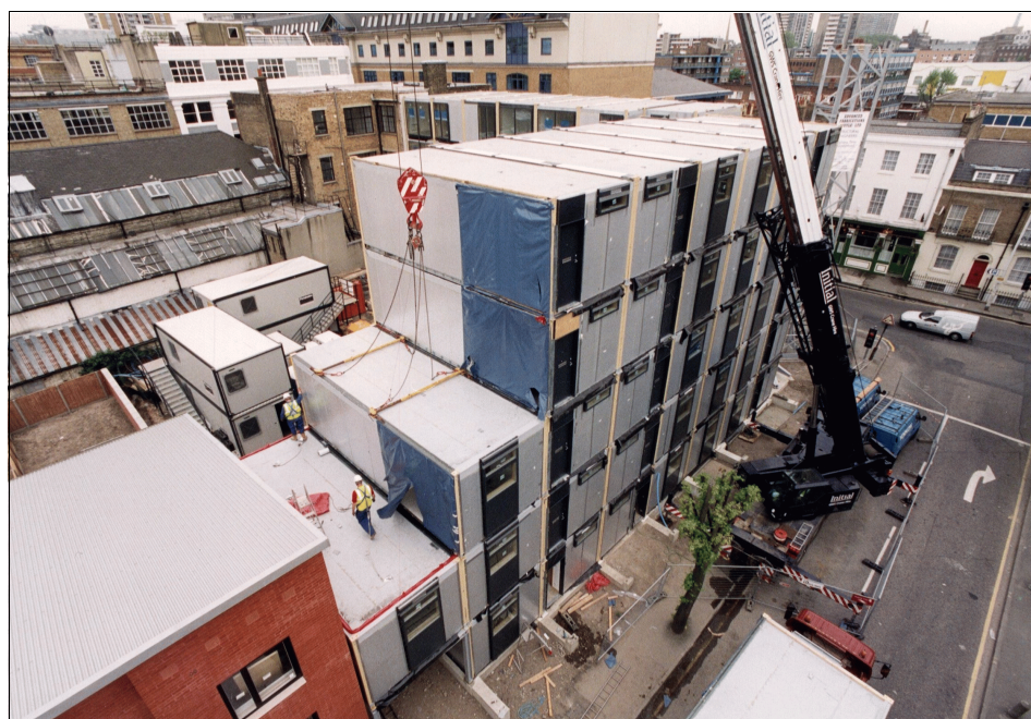
Figure 1.5 Installation of modules at Murray Grove, Hackney, London
