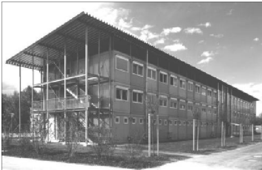
Figure 5.5 Relocatable office building for a local authority in Munich
