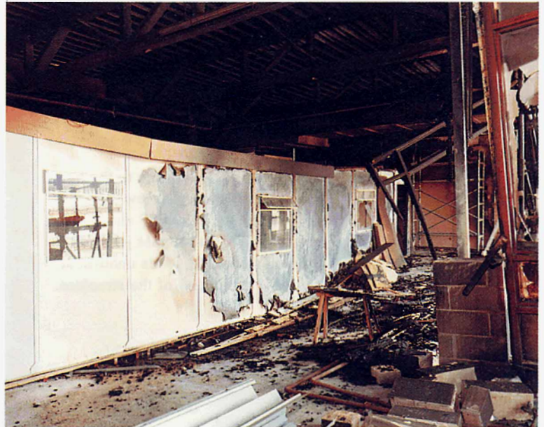
Plate 2: Photograph of a sub-contractor's hut typical of that which was destroyed during the fire. This hut is located at Level Two and was damaged externally during the fire as a consequence of flames through the windows from the fire at the floor below. Note flaking pvc wall coating.
