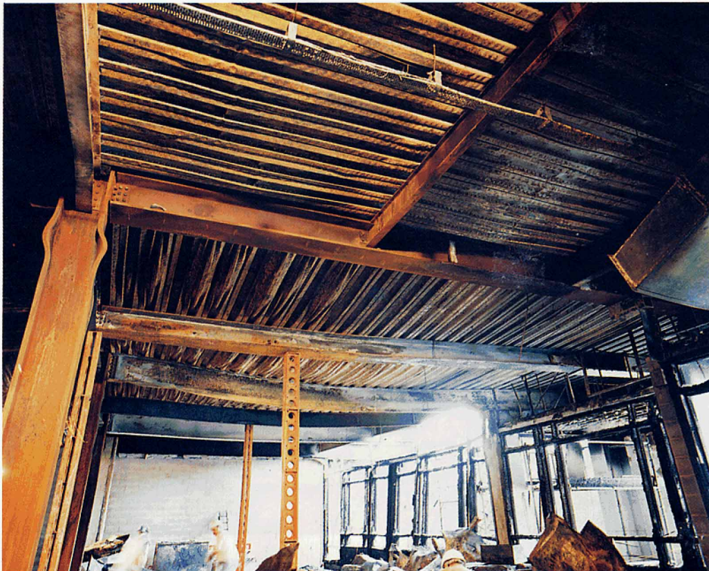
Plate 10: View towards Phase 7 and Exchange Square showing column C34.
