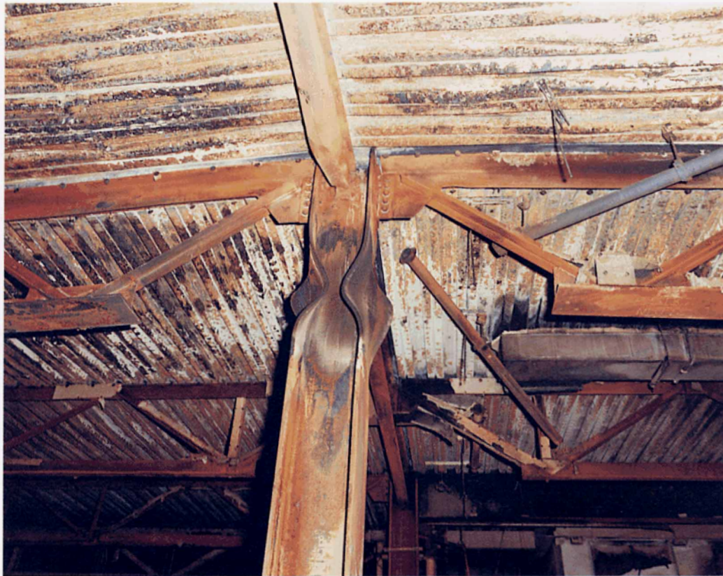
Plate 12: View towards Phase 7 of Column E33
