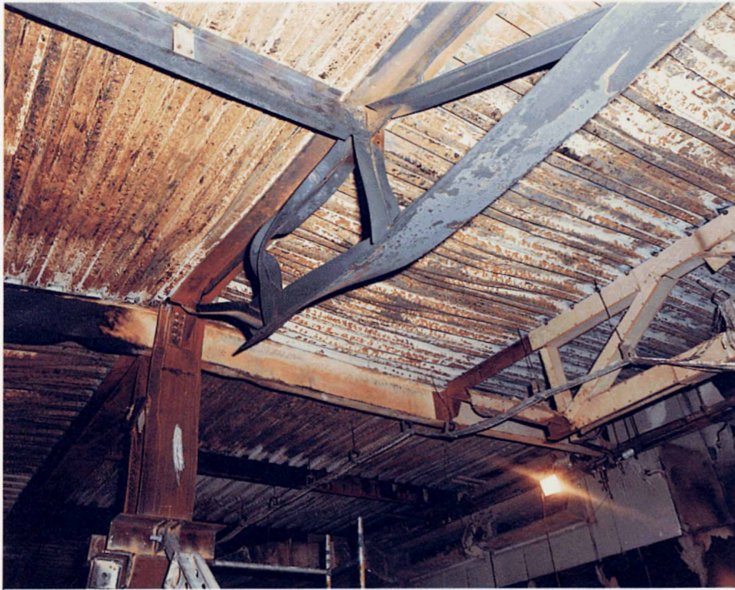
Plate 11: View towards Exchange Square showing column C34.
