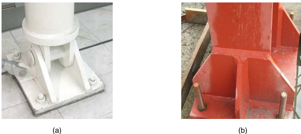
Figure 2.3 (a) Nominally pinned column base and (b) rigid column base with stiffeners
