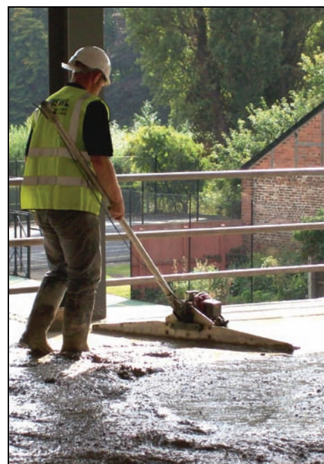
Concrete surface floated smooth
