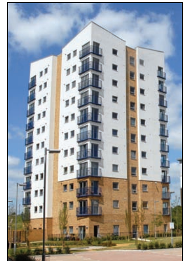
11 storey modular block
