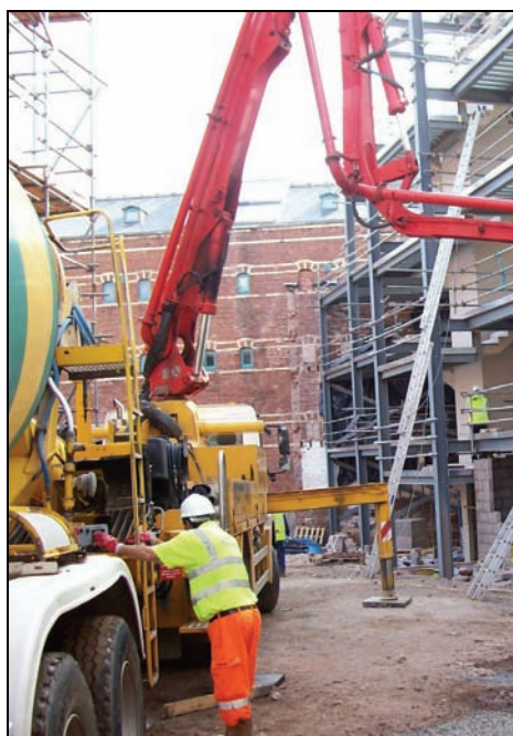
Concrete pumped onto decking
