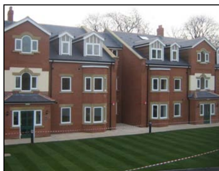
Broomlands Development in Middlesbrough using light steel framing
