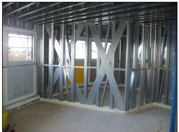
Braced walls in load bearing structure
