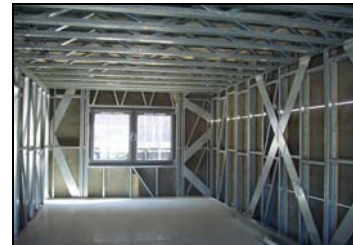
Light steel framing system
