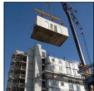
Module during construction
