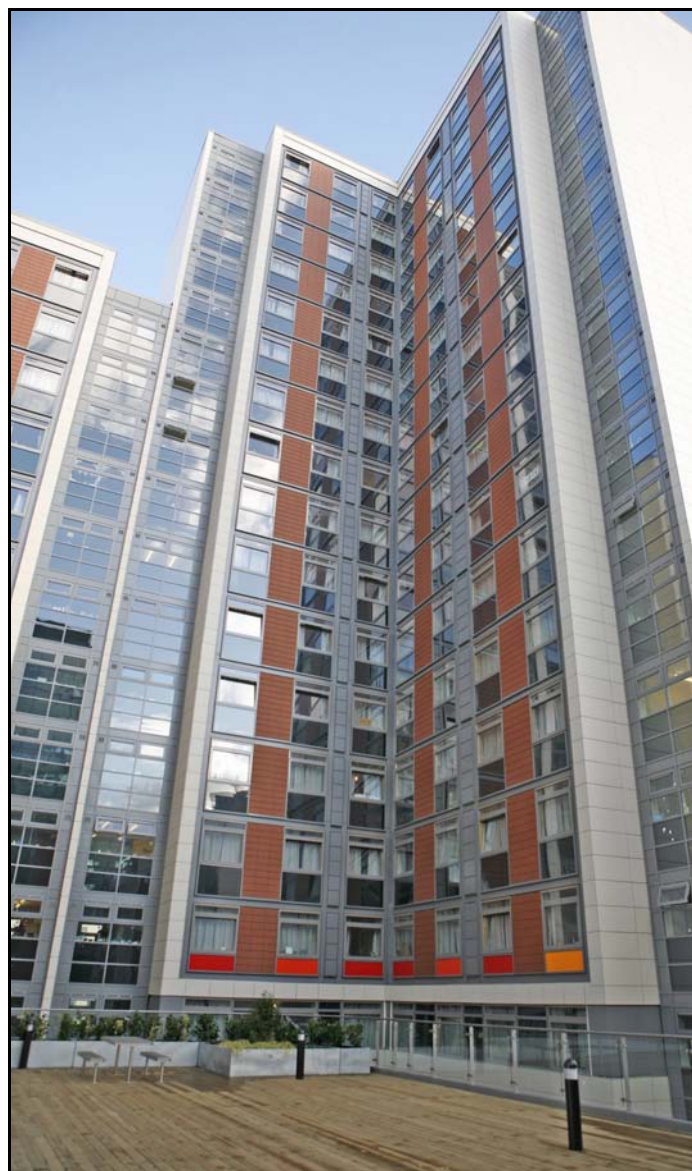
Seventeen storey modular building at Paragon project
