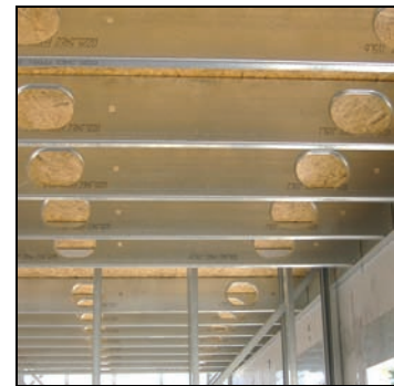
Light steel joist
