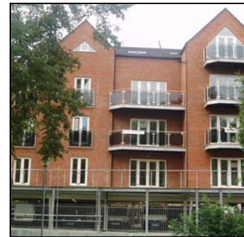
Car park below apartments
