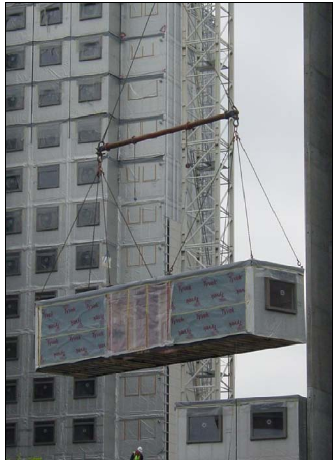
Lifting an open-sided module
