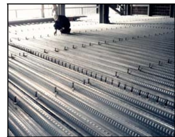
Composite deck on steel beams
