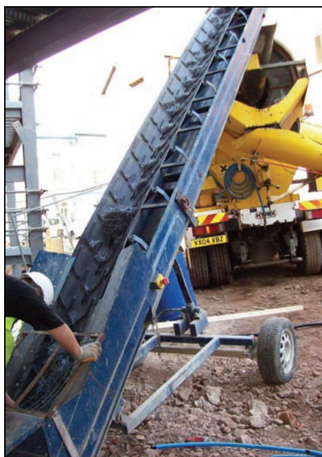
Fibres added to concrete mix
