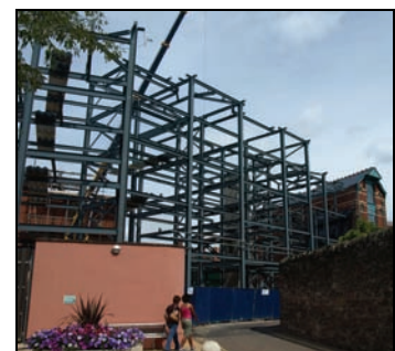
Structural steel frame
