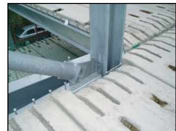
Hollow core units on steel frame
