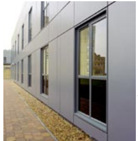
Steel cassette attached to light steel frame
