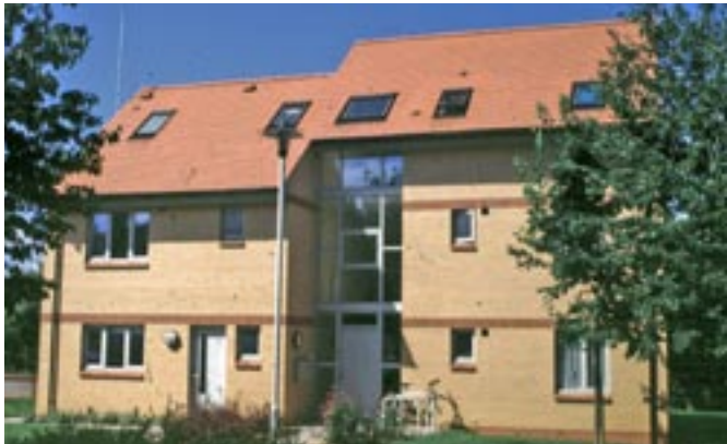
Finished building at Oxford Brookes University used for long term monitoring
