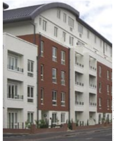
Insulated render attached to light steel frame
