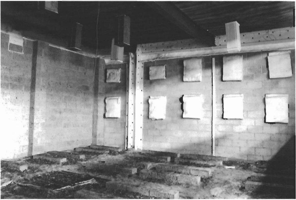
Figure 6.18 Internal view of compartment (looking towards gable wall) following the test
