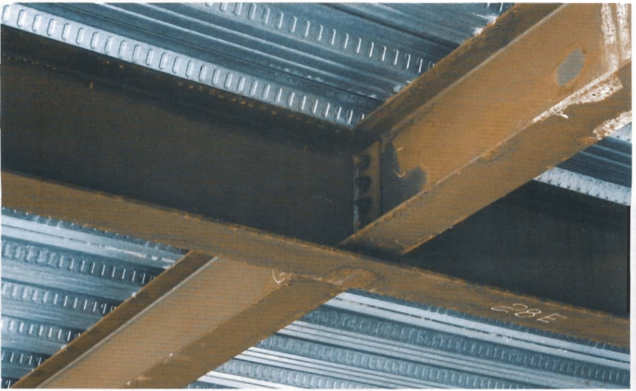
Figure 5.4 Fin-plate (beam-to-beam) connection
