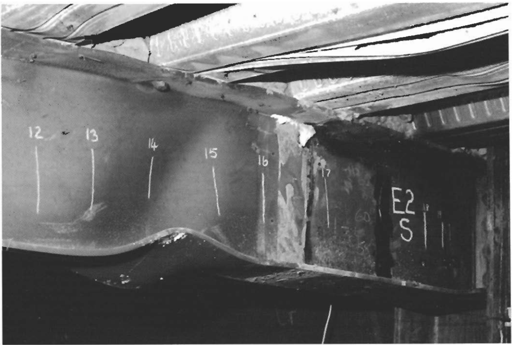
Figure 6.4 Test 1: Local buckling of test beam just inside furnace
