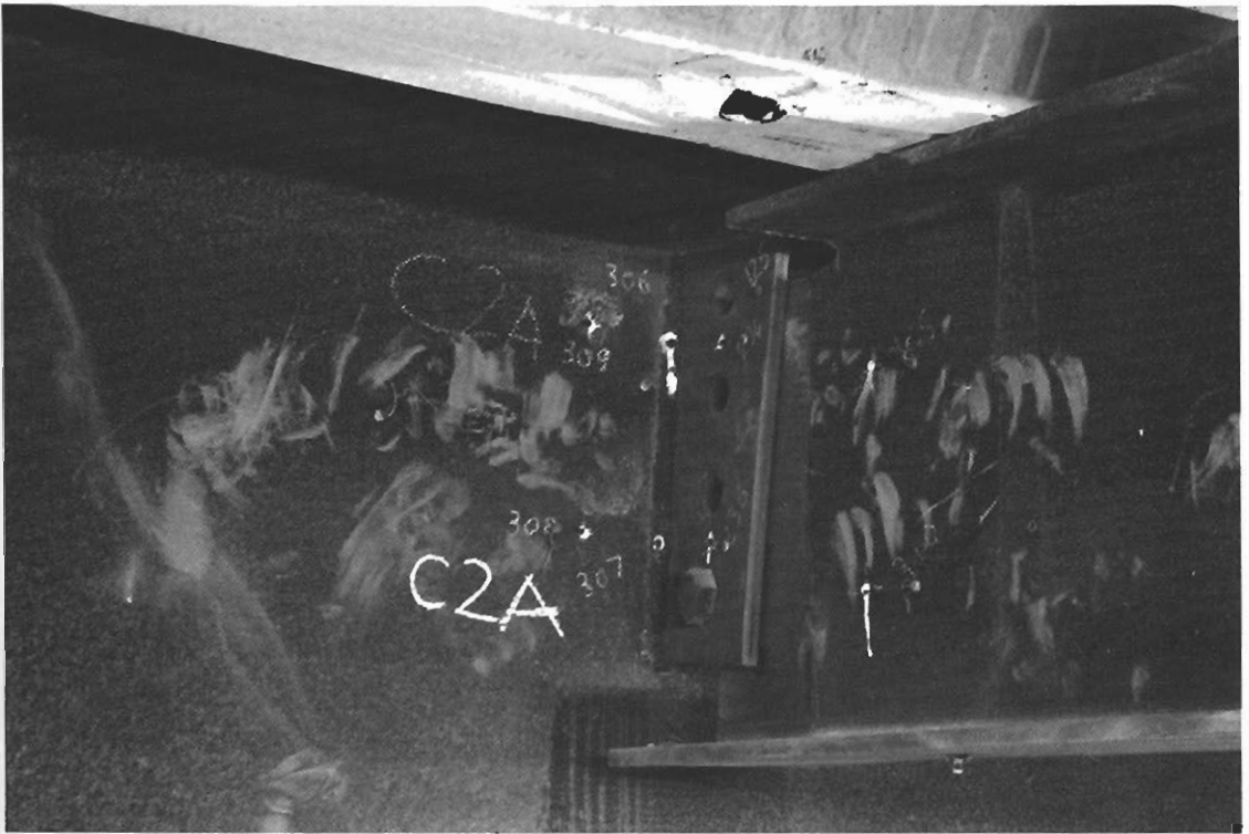
Figure 6.12 Bolt shear in beam-to-beam connections (fin-plates)
