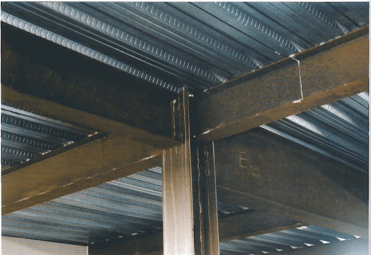
Figure 5.5 Flexible end-plate (beam-to-column) connection
