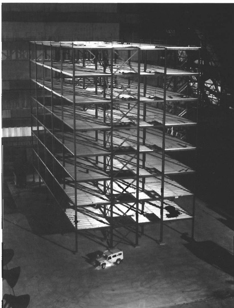
Figure 5.1 General view of the structural frame
