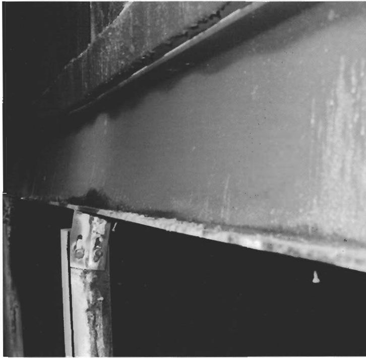
Figure 6.22 Twisting of external beam to external beam
