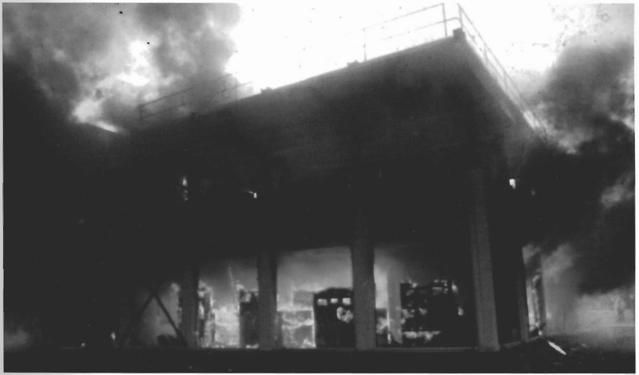
Figure 3.2 BHP fire test
