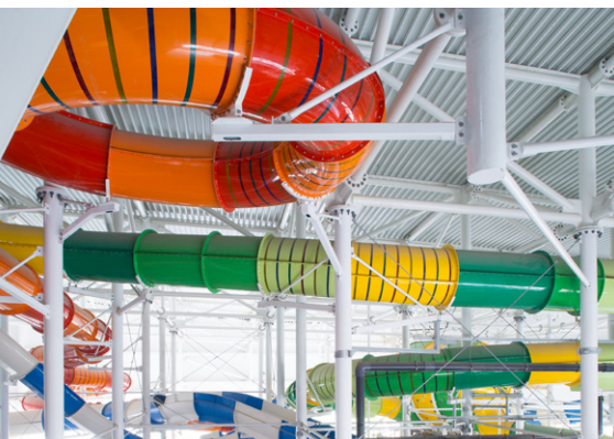
© Billington Structures Ltd
