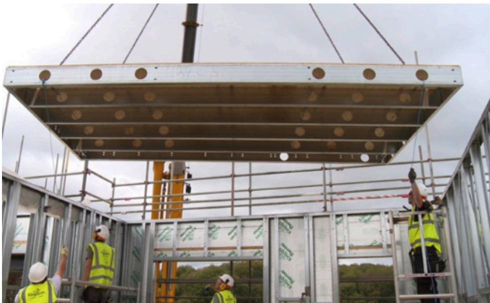
Typical light gauge floor cassette
