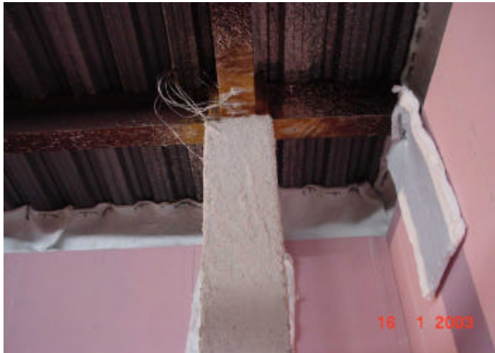
Figure 6 Internal column (D2) protection to underside of connecting beams
