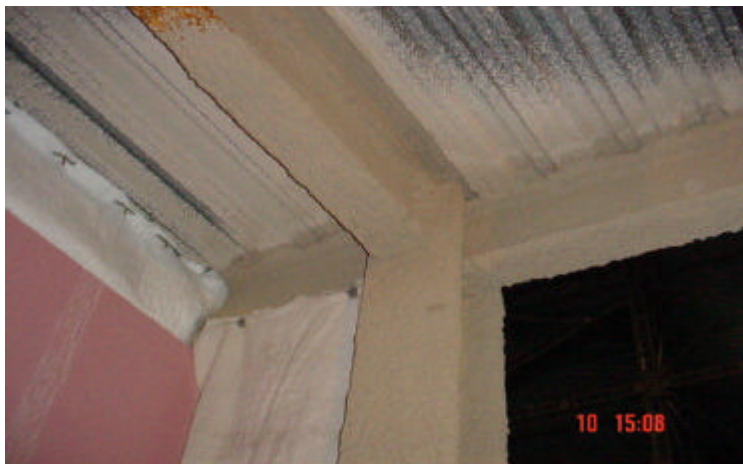
Figure 7 Perimeter column protection including connections and “coatback” length
