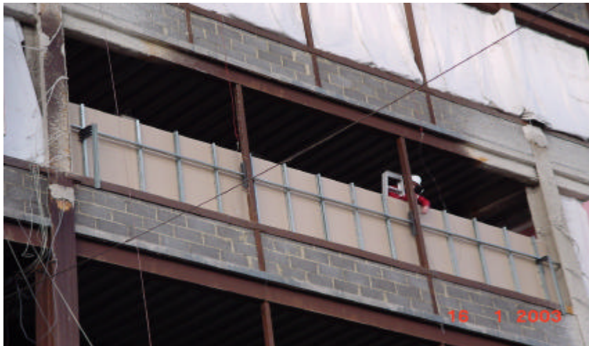
Figure 3 Fireline plasterboard over window opening
