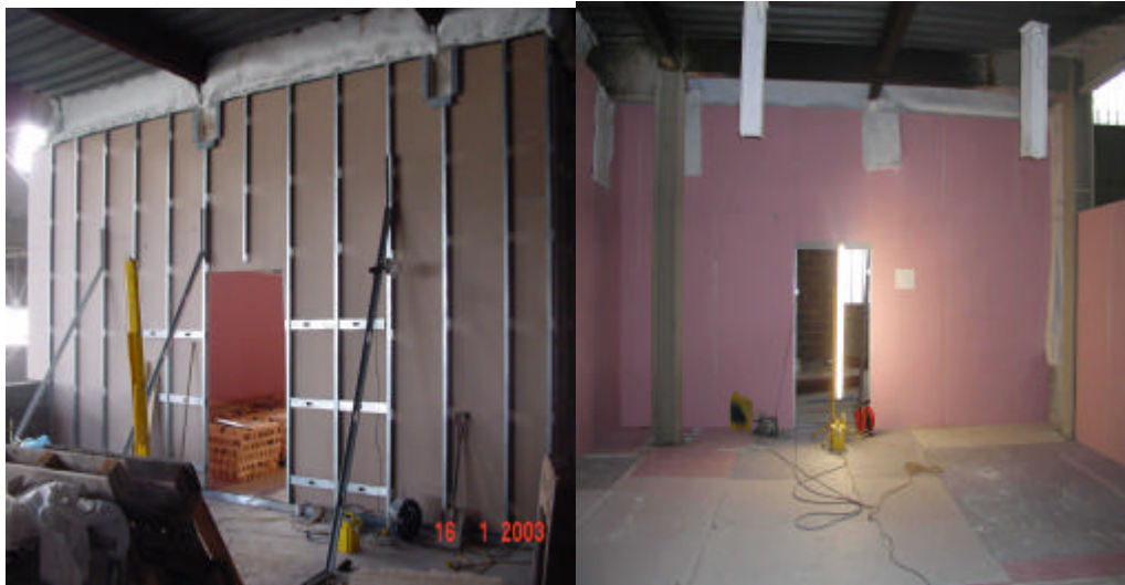
Figure 2 Compartment wall parallel to gridline E – external and internal view
