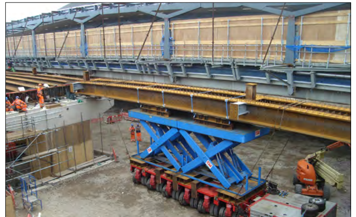
Ingenious: Cleveland Bridge has developed a special method of erecting girders
