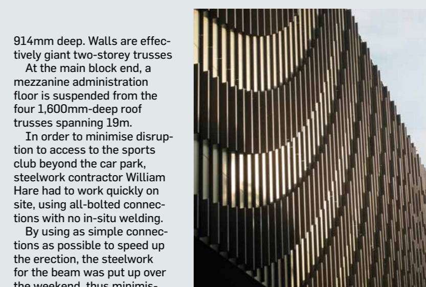
Left: Perpendicular aluminium fins on the sports beam elevations create a pattern inspired by Newton's rings. Right: The sports beam was erected swiftly, supported by five sets of paired columns.
