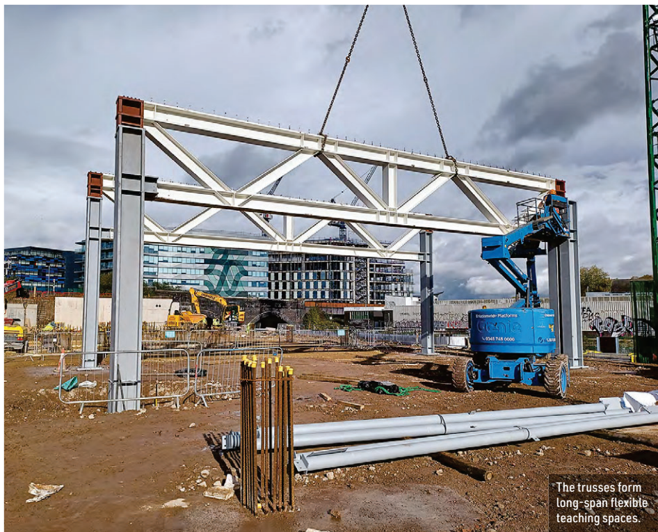
Two trusses, which are not connected, are positioned either side of a movement joint.
