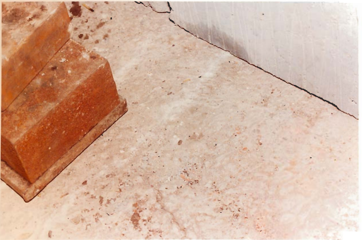
CONCRETE SLAB AFTER TEST SHOWING CRACKING IN THE CENTRE AND AT THE ENDS FIGURE 12.
