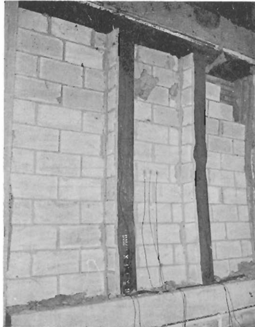
356 x 171 mm x 67 kg/m BEAMS IN WALLS CONSTRUCTION AFTER TESTING
