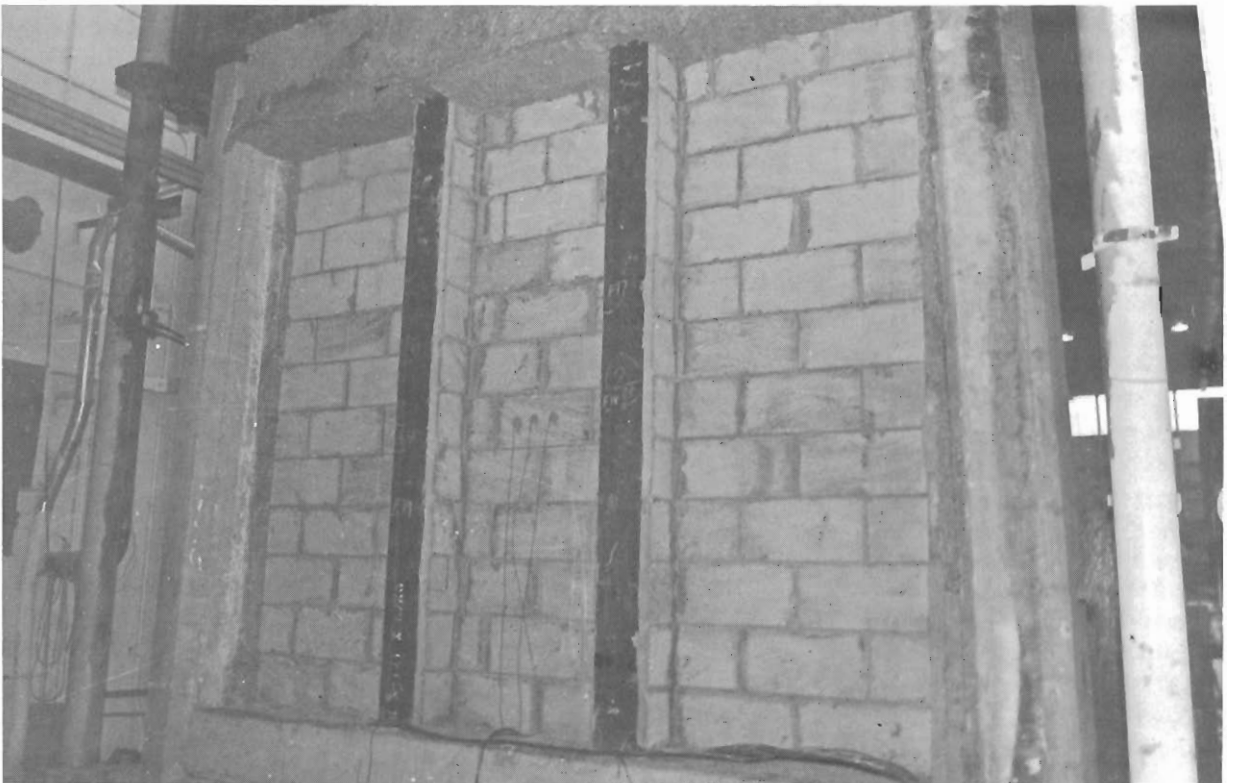
356 x 171 mm x 67 kg/m BEAMS IN WALLS CONSTRUCTION PRIOR TO TESTING
