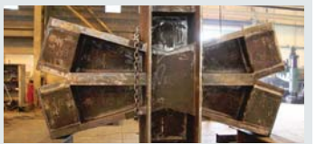
One of the complex steel nodes, constructed off site.
