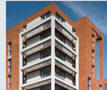
Fully glazed communal areas are positioned on the corner, with balconies expressed in white render in contrast to the brickwork.
