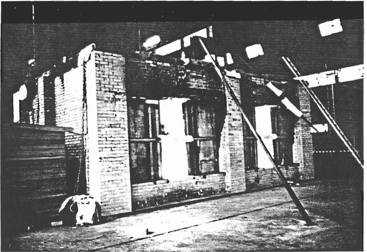
FIRE TEST IN PROGRESS FIG. 9
