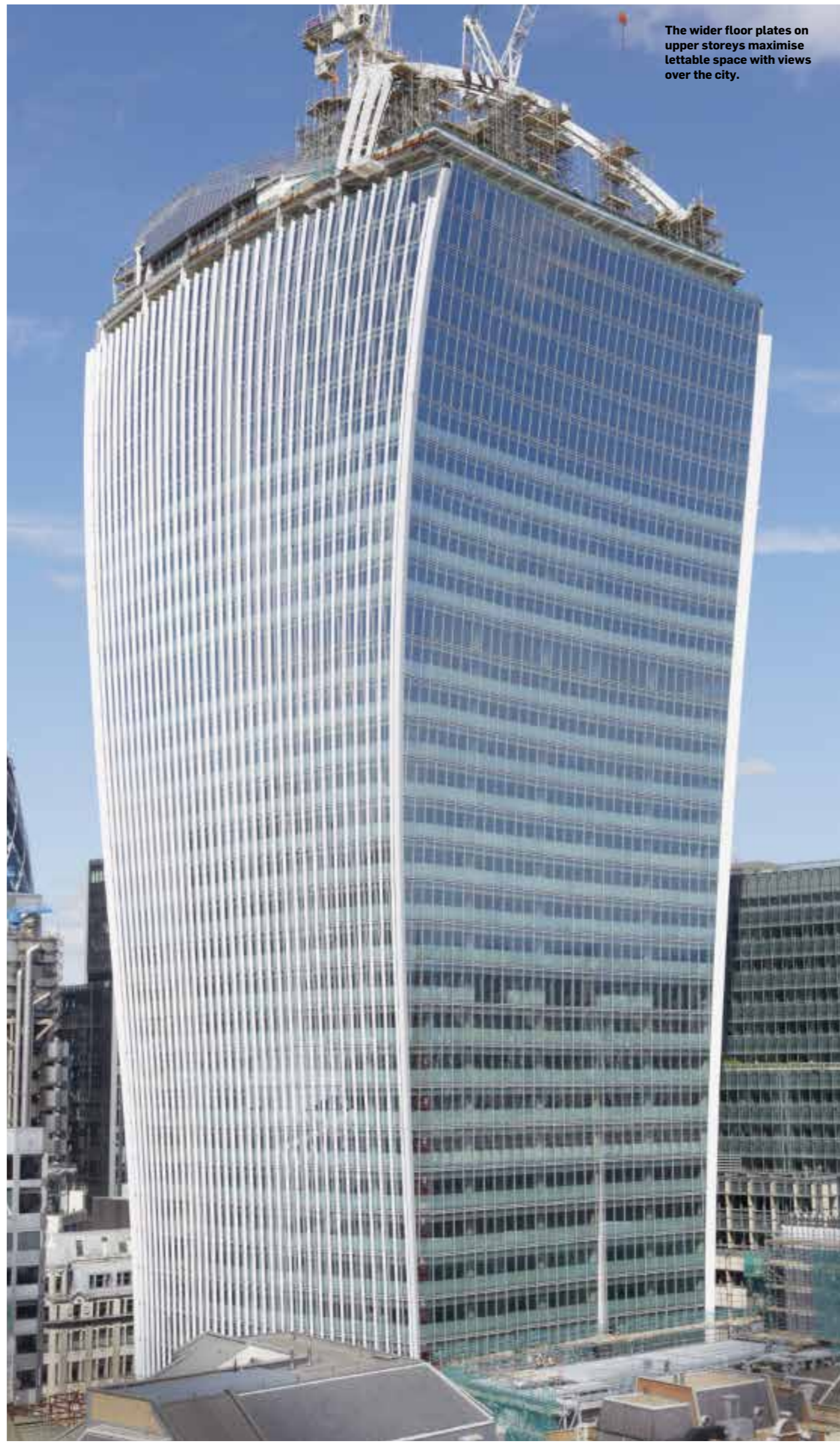
North section: 20 Fenchurch Street's pint-glass profile is created as the floor plate flares and then tapers back on the upper storeys.
