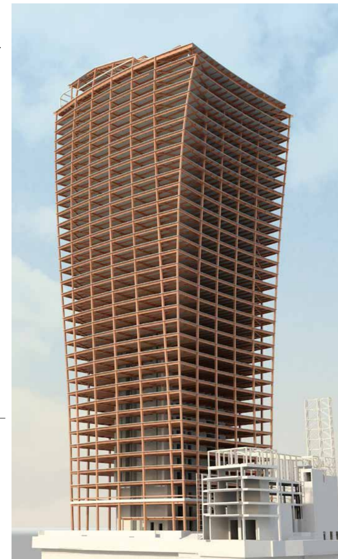
The steel frame is made up of approximately 8,500 major structural members.
