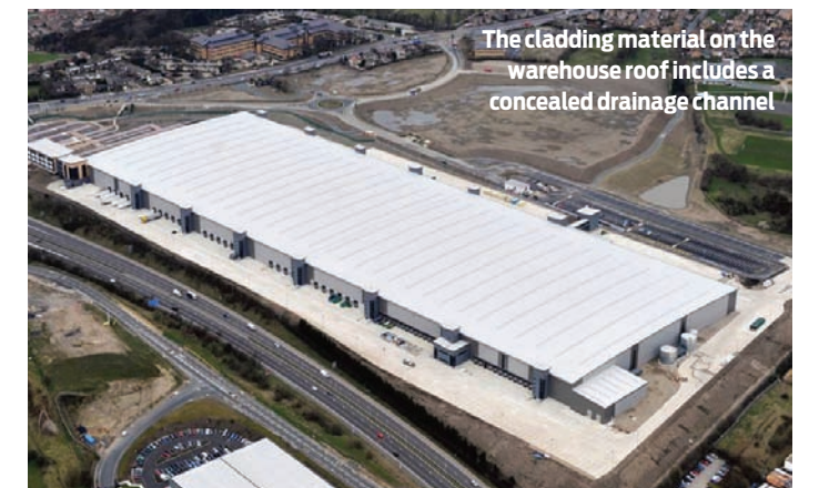
Erection of this Marks & Spencer warehouse in Bradford used 3,000 tonnes of steel and took just 12 weeks
