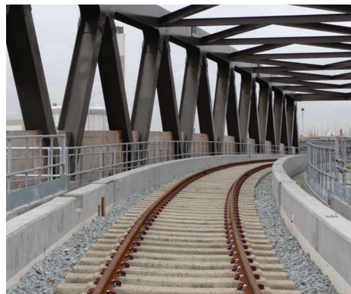
The 690-tonne steel structure is 75 m long and 8 m deep, and was installed in 2008 during a planned closure of the line
