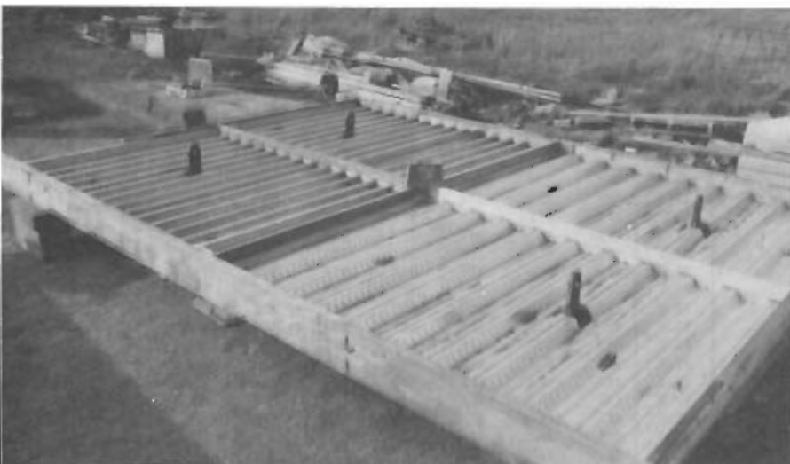
Orientation of deck span to beams (c)
