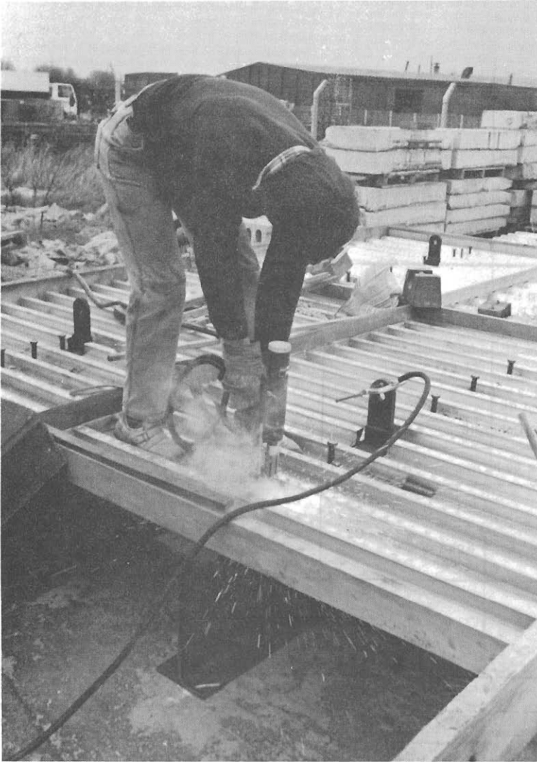
STUD WELDING SHEAR CONNECTORS
