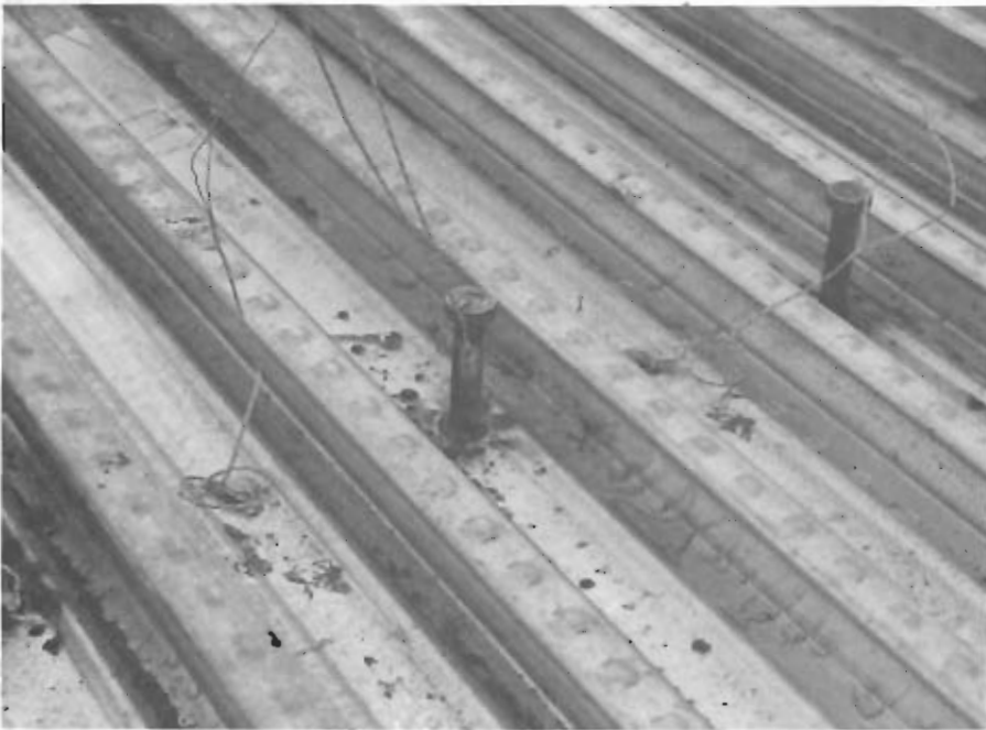
Thermocouples attached to shear studs (b)
