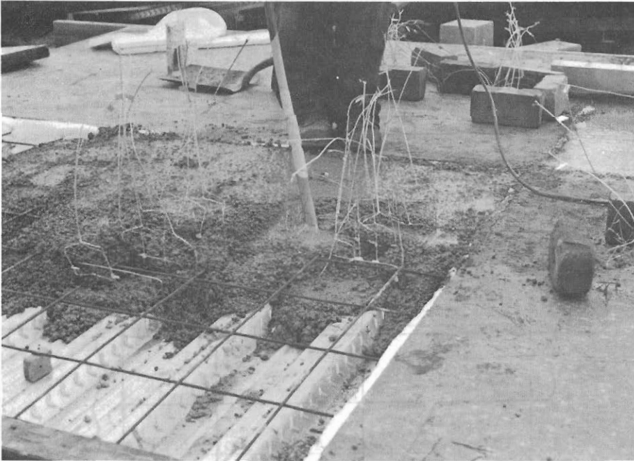
POSITIONING OF THERMOCOUPLES WITHIN THE CONCRETE
