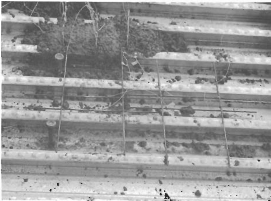
POSITION OF ADDITIONAL REINFORCEMENT MESH
