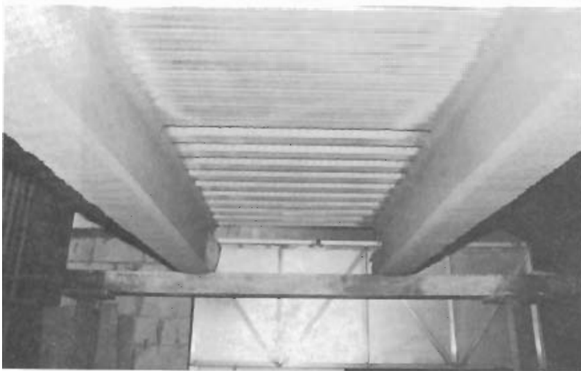
(a) Beams protected with Mandolite P20
